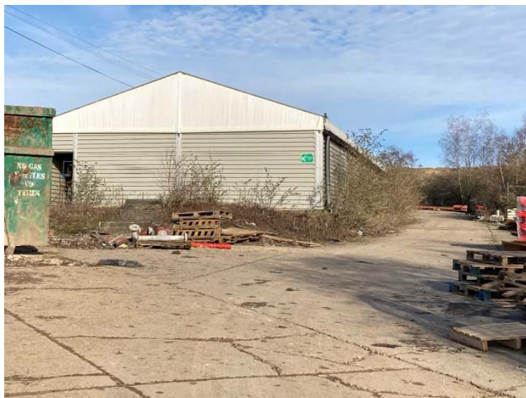
Plate 7. Building 1 in the south-east of the Site
