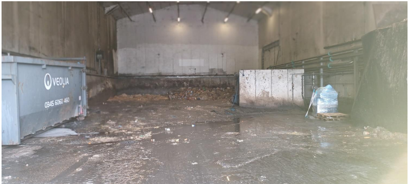
Photograph 3: Waste reception building before improvement work
