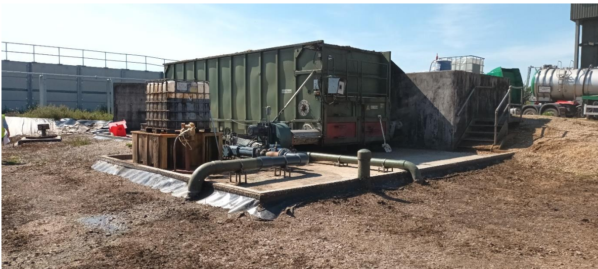
Photograph 6: Crop feeder for digester 1 with banded storage for IBC (redundant)
