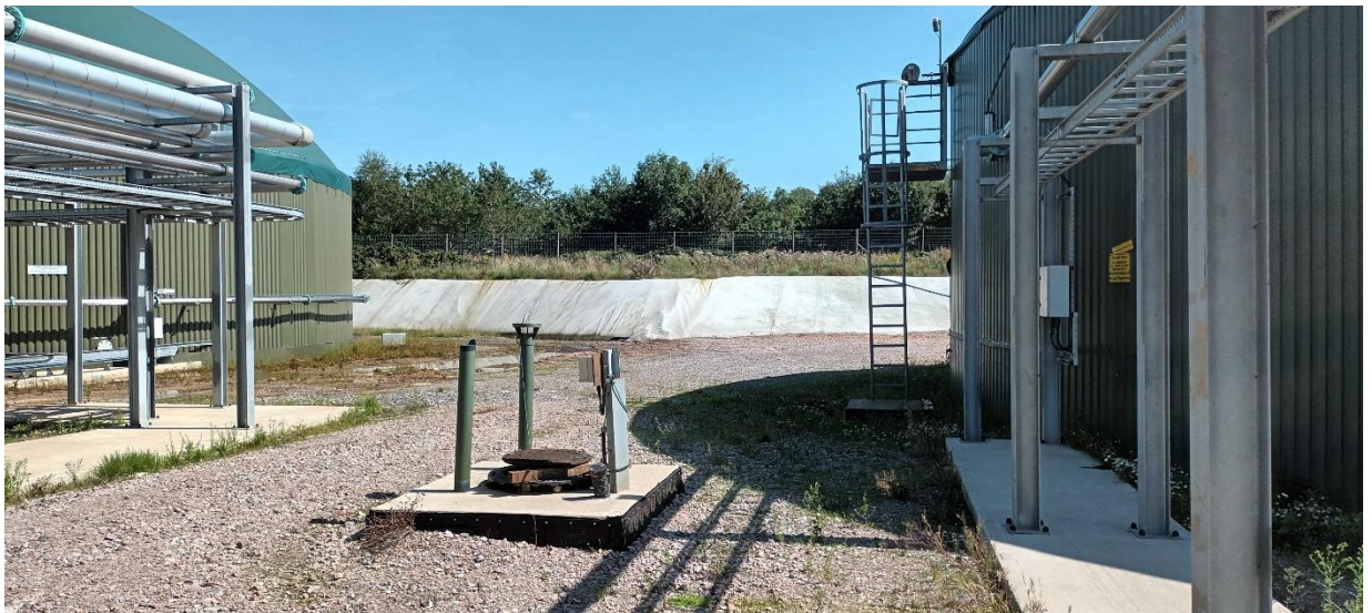
Photograph 16: Area between D2 and Post Digester looking northeast
