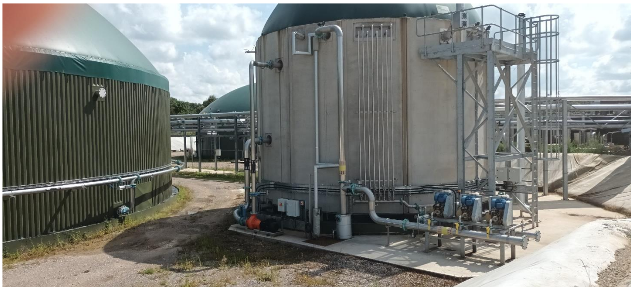
Photograph 23: 3 No. new tanks within containment area
