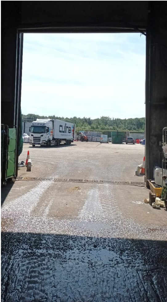
Photograph 5: Concrete apron to south of waste reception building
