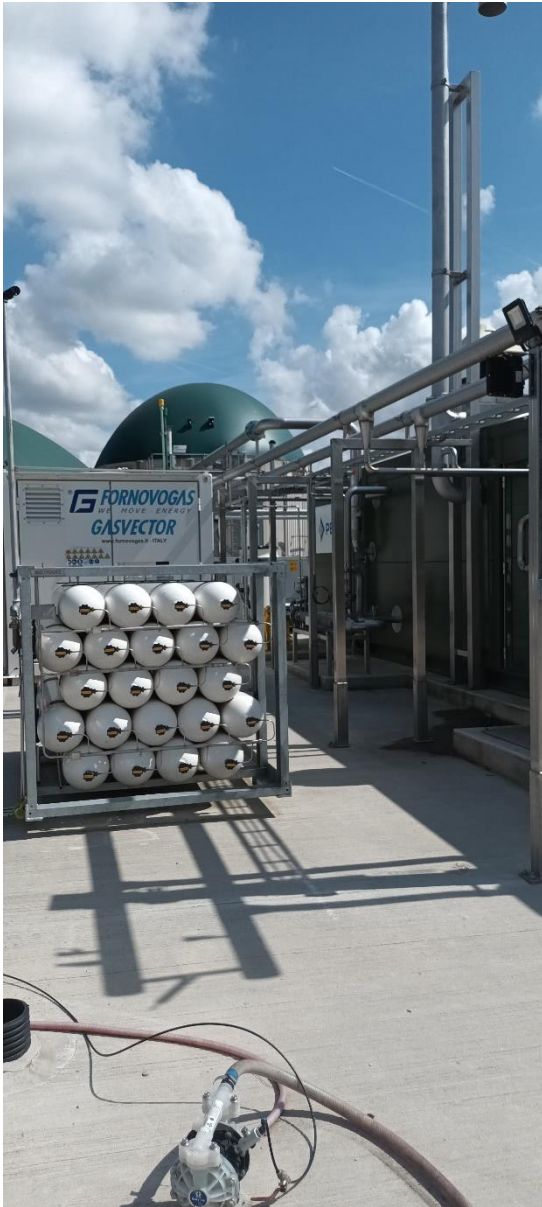
Photograph 20: Biomethane storage for refuelling
