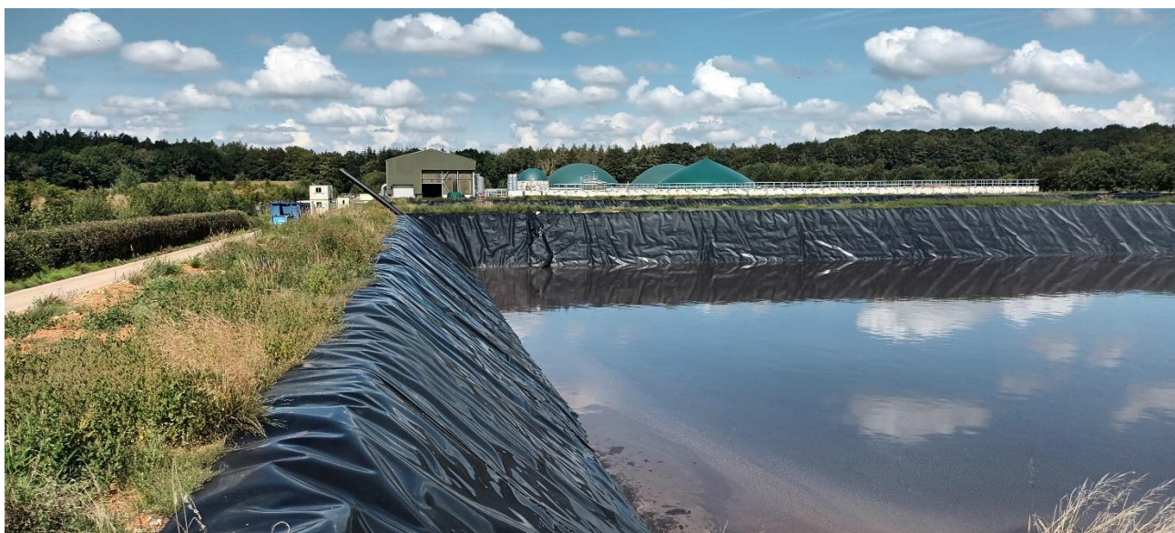
Photograph 24: New digestate storage lagoon (south lagoon)
