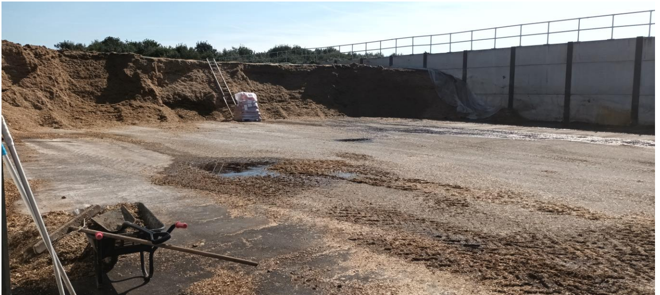
Photograph 1: Silage clamp surface (prior to improvement work)
