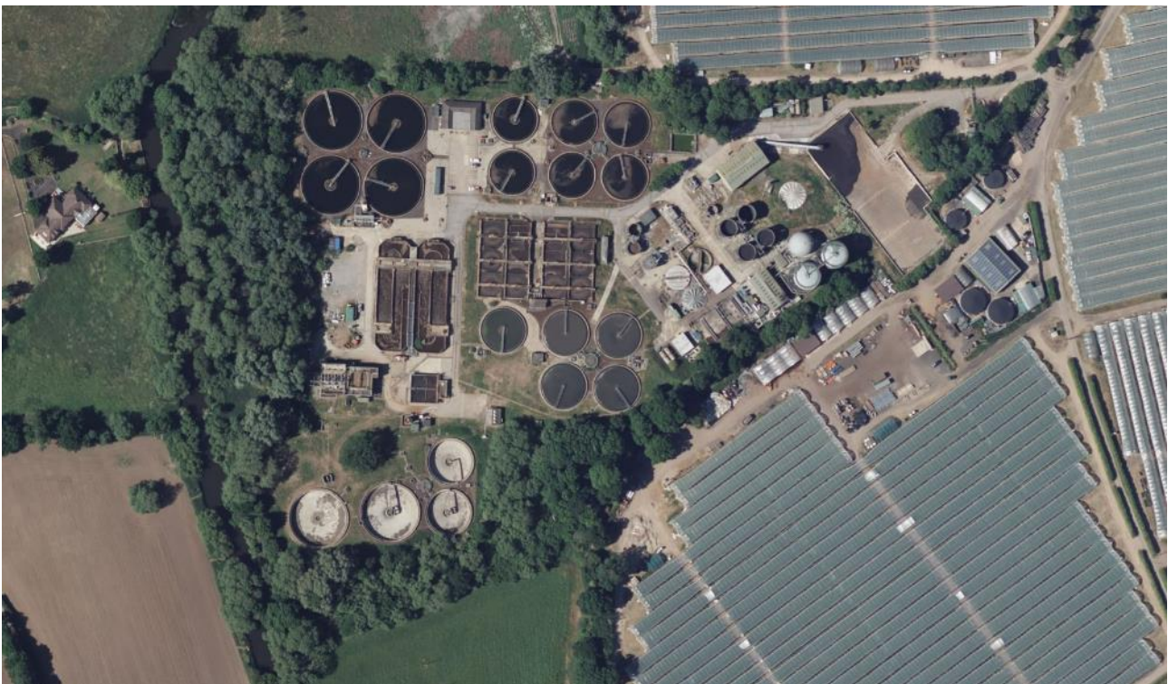
Figure 2-2 - Satellite view of Wargrave Sewage Treatment Works
