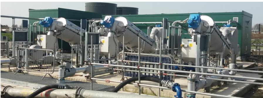
Photo 1 – Drum thickeners (x3)
