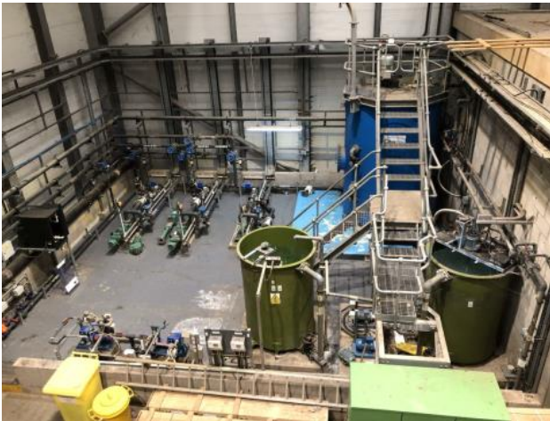
Photo 15 – Polyelectrolyte preparation area
