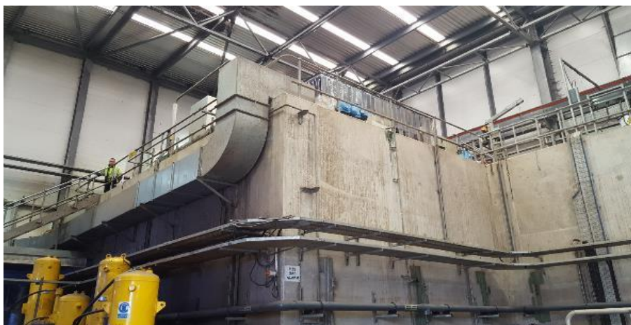
Photo 6 – GBTs within the building
