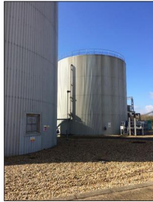
Figure 10: Primary digester
