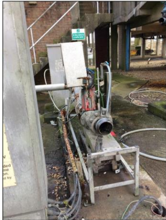
Figure 7: Cess inlet connection
