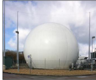
Figure 15: Double membrane gas bag
