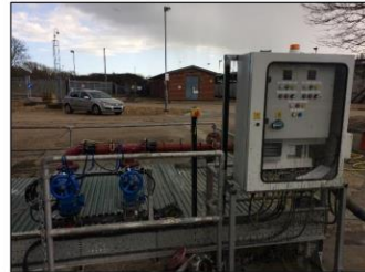
Figure 5: Commercial waste pumping section
