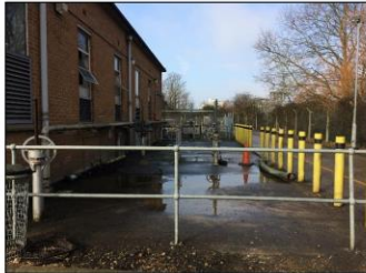
Figure 1: PS3 underground wet well / inlet works.
