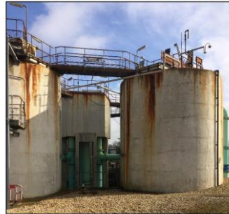
Figure 3: Inlet 2 (Portsmouth catchment)
