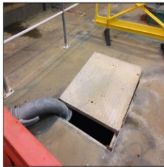
Figure 3: Open hatch to inlet works.
