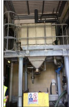
Figure 5: Cess settling tank / hopper.
