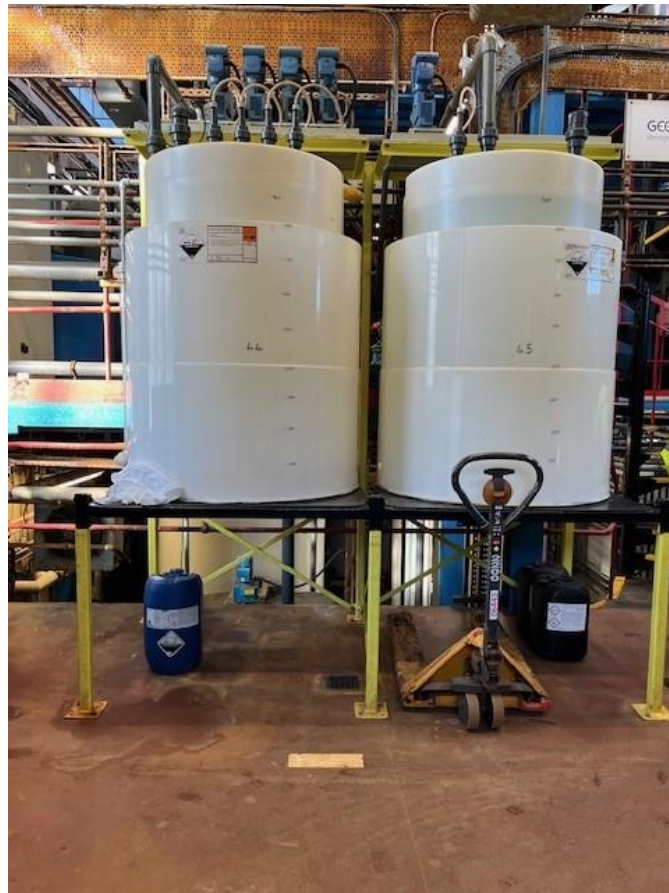
Fig 11 – Bunded chemical dosing tanks within the ETP.
