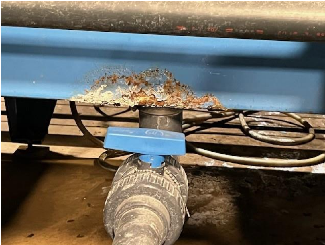
Fig 5 – Corrosion damage at exit manifold from Cleaning bay tank A13.
