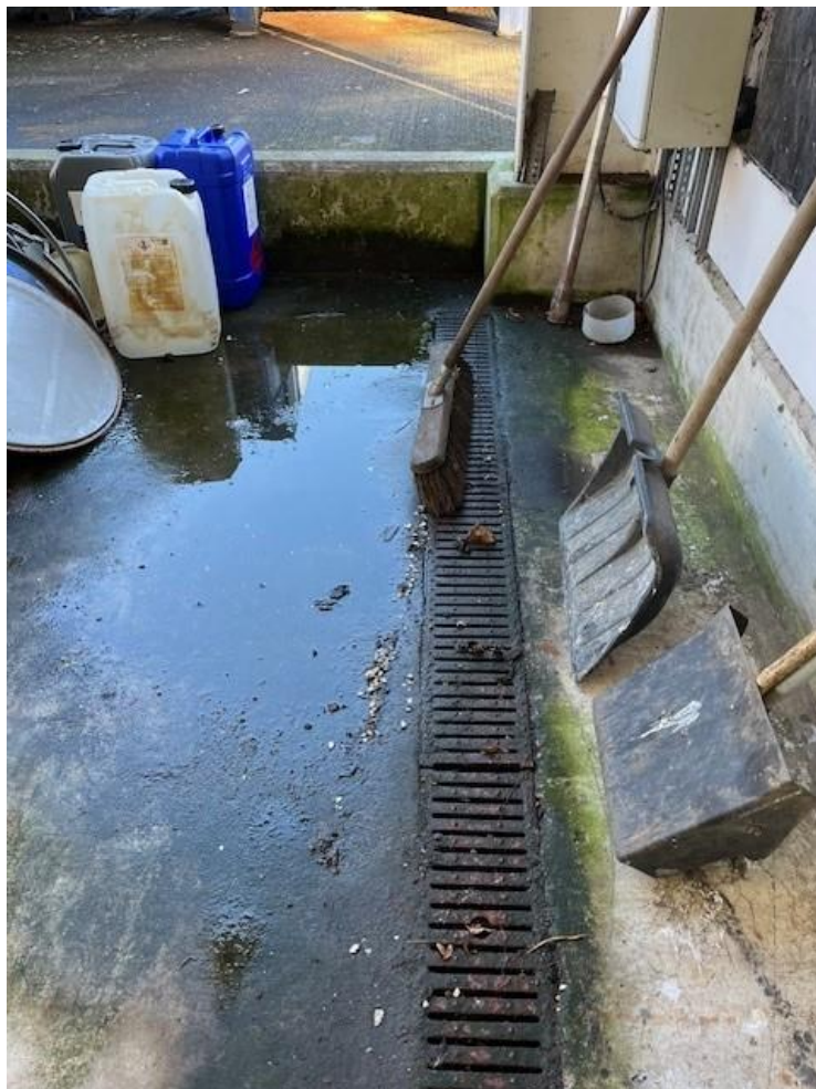
Fig 16 – Sealed channel drain at rear of MRF.
