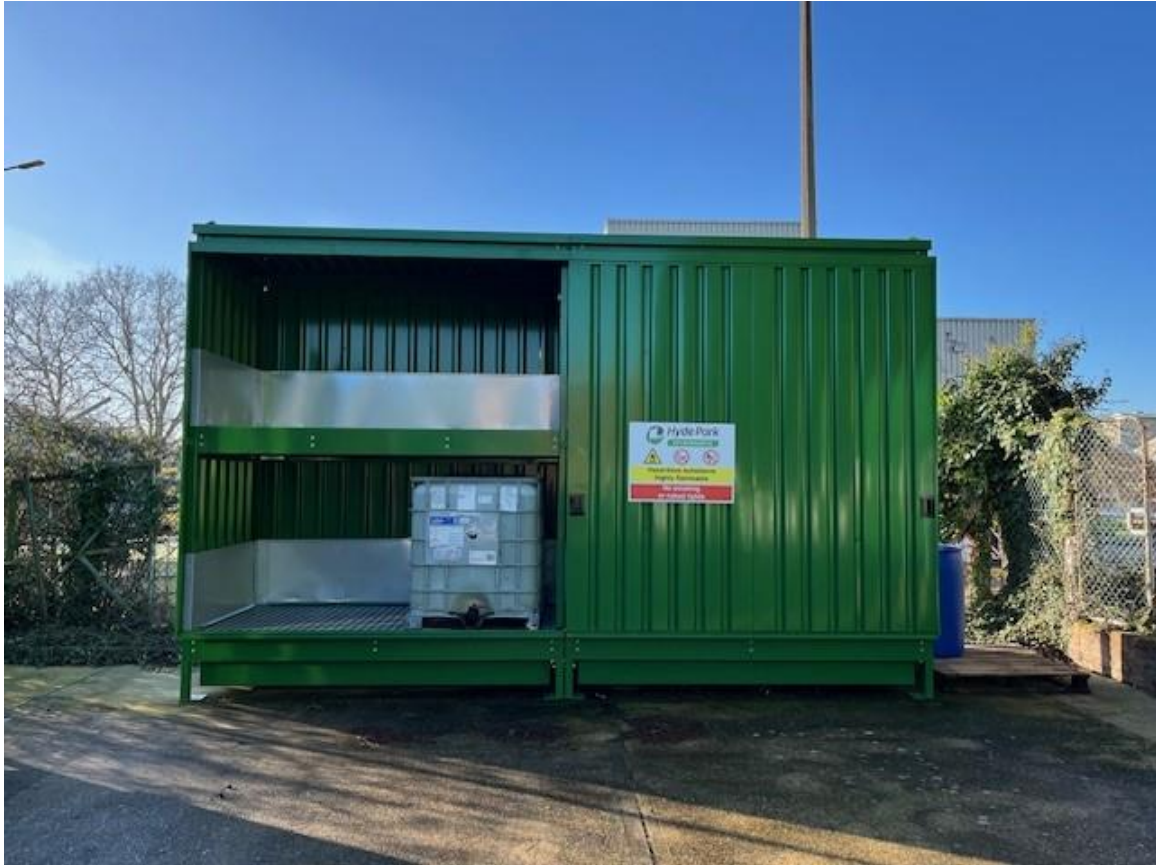
Fig 1 – New bunded liquid chemicals storage bay adjacent Building 99.
