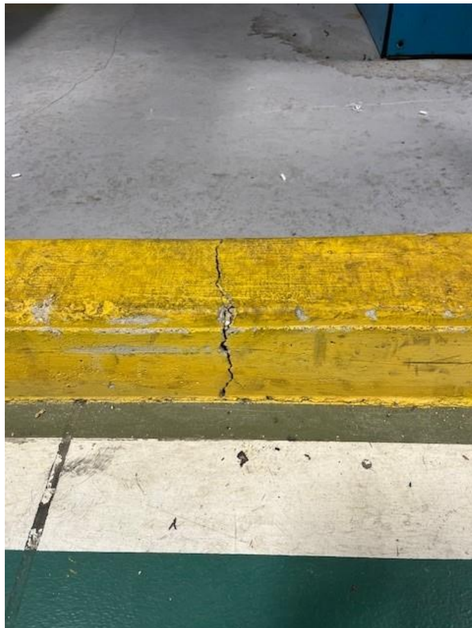
Fig 6 - Cracked peripheral concrete bund at front of spray booths area.
