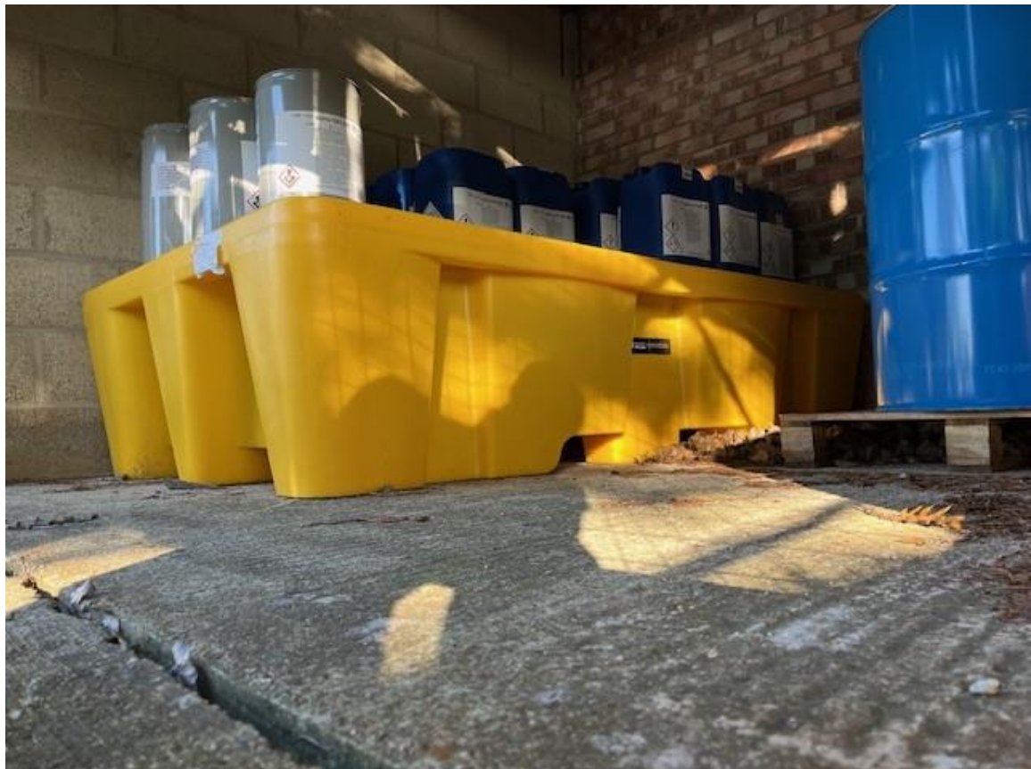
Fig 2 – Bunded storage area for dry chemicals adjacent Building 99.
