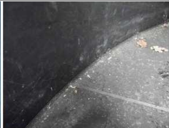
Photograph 15: Bund floor to shell internal corner weld in good condition
