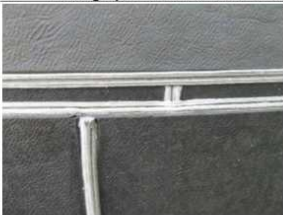
Photograph 12: External bund is in good condition. Welds all good.
