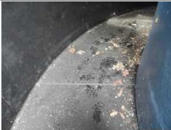
Photograph 14: The tank bund bottom was relatively clean and dry.
