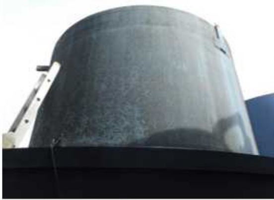
Photograph 1: Tank is on stream with no permanent access.
