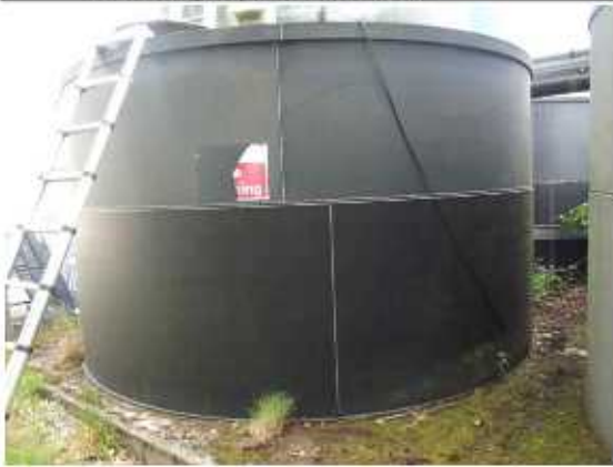
Photograph 3: Tank foundation is cast concrete slab construction.
