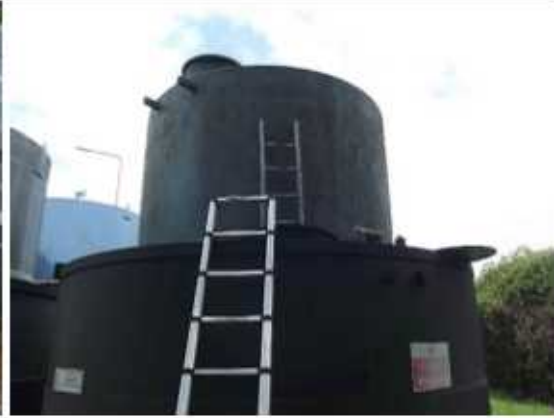
Photograph 2: Manway is in the bund lid. Temporary ladder access.
