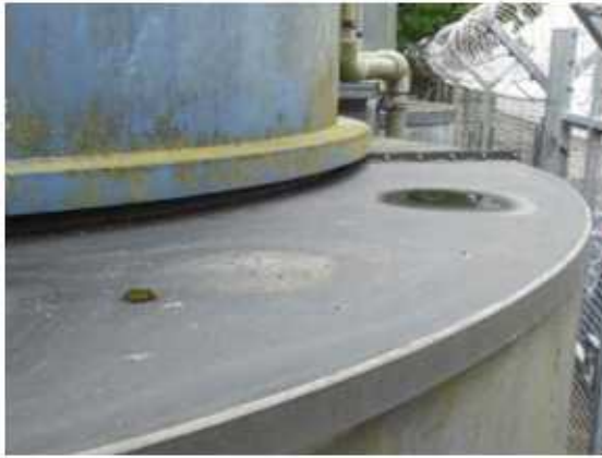
Photograph 15: Bund lid below steel rainwater deflector skirt.
