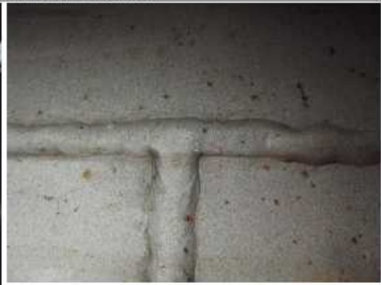
Photograph 11: single horizontal and vertical weld over two courses.
