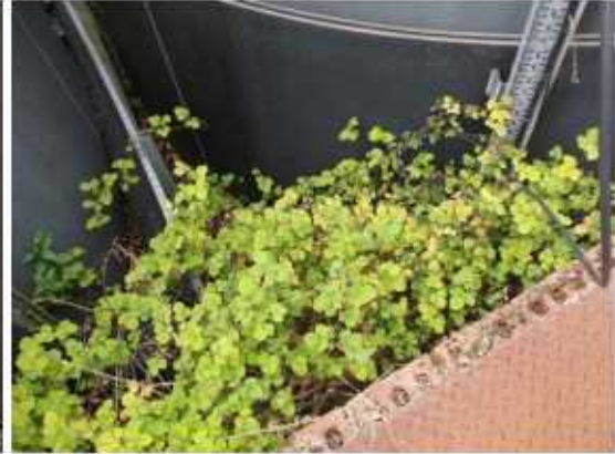
Photograph 7: Significant vegetation in and around tank bunds.
