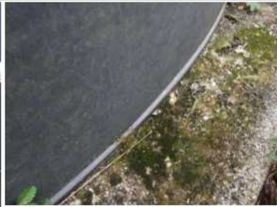
Photograph 4: Tank bund is installed directly on top of the foundation.
