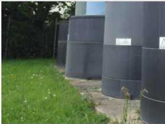
Photograph 3: Tank foundation is cast concrete slab construction.
