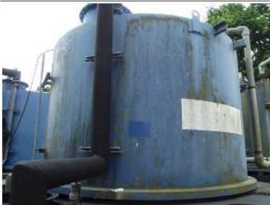
Photograph 8: The tank shell above the bund is in good condition – painted blue..
