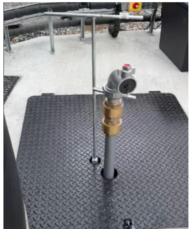
Purpose built discharge point
