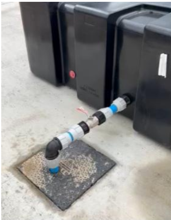
Discharge point to foul sewer
