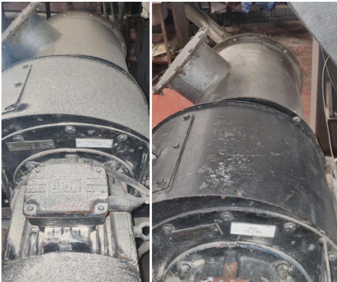
Figure A5 - dust levels on FD fan shortly after clean ( boiler 5 on left, boiler 4 on right)
