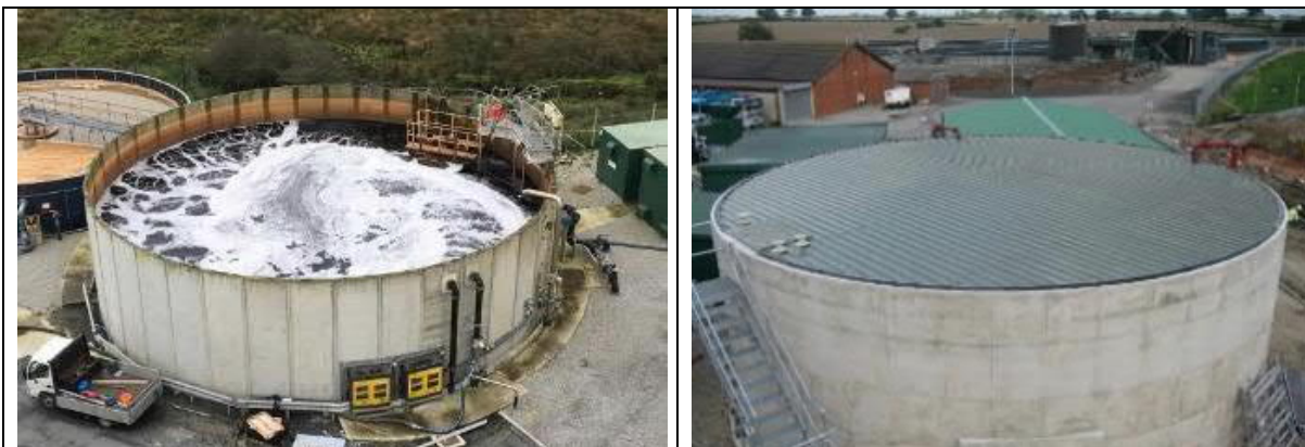
Figure 2-4 – BT 2 Before and After Installation of Cover
