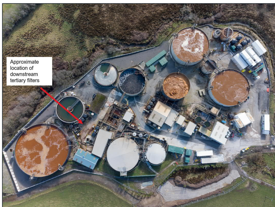
Figure 4-29 – Downstream Tertiary Filters Location
