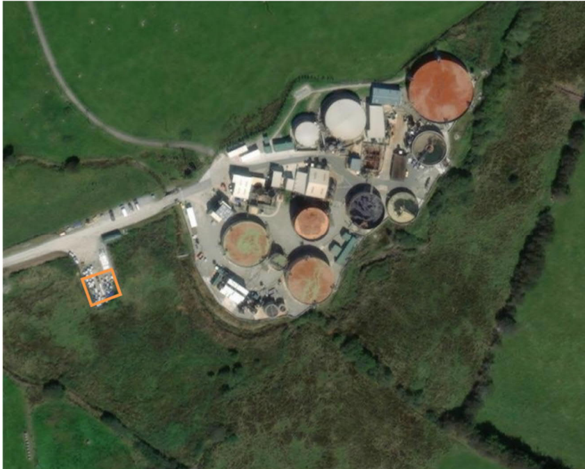
Figure 4-2 - Site of Chemical Storage Area
