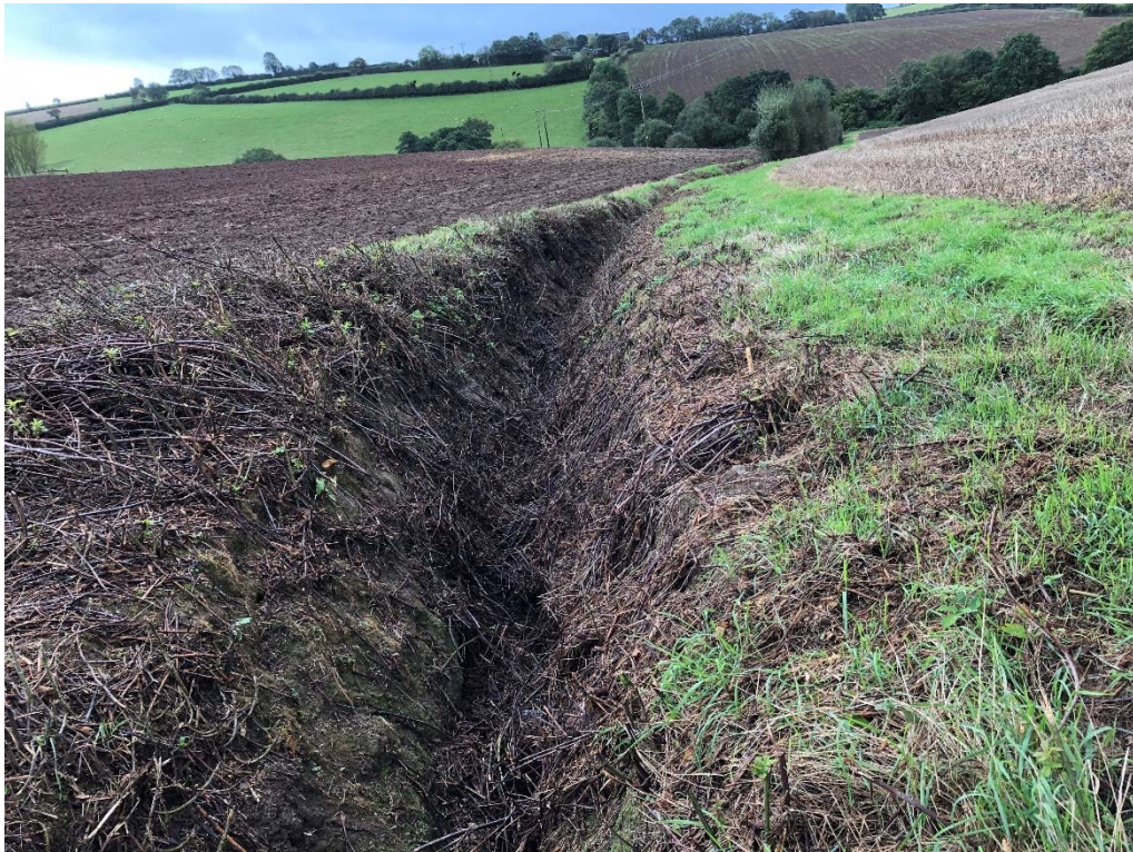
Photograph 17: Surface water ditch heading in a southerly direction towards unnamed water course to south of Site. Ditch observed to have been cleared subsequent to 20 August 2019 walkover. Ditch dry adjacent to deposition area despite heavy rainfall in period prior to walkover survey. [01 October 2019].
