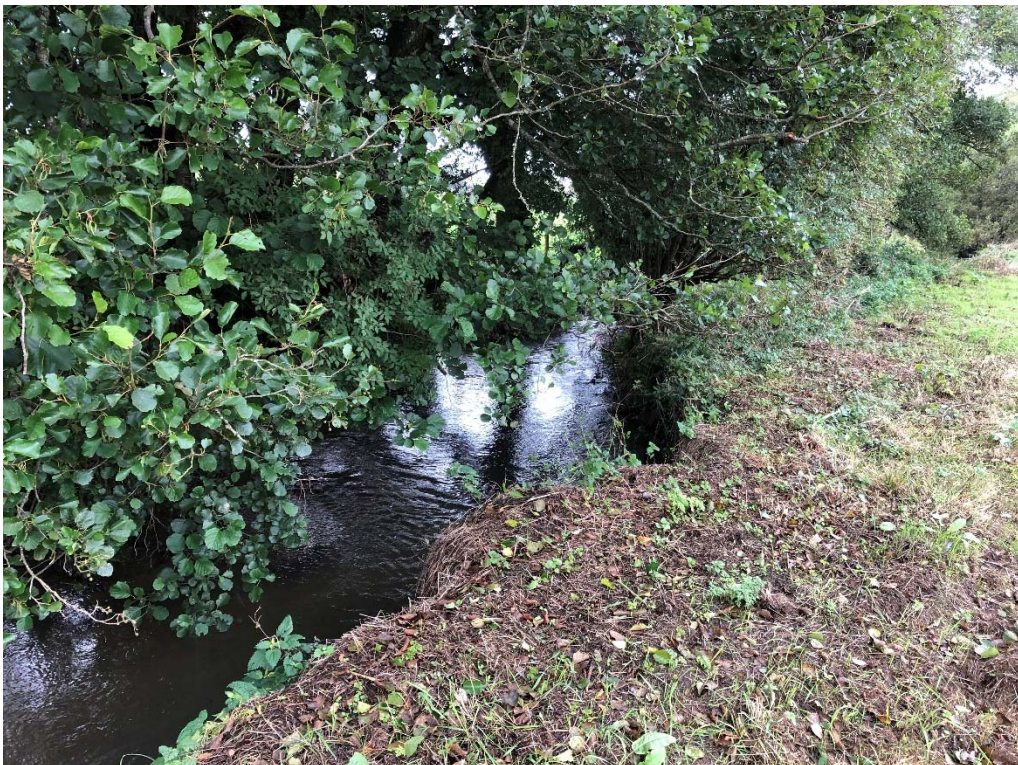
Photograph 22: Unnamed water course to south of Site, looking in a westerly direction upstream of point where surface water discharges. [01 October 2019].
