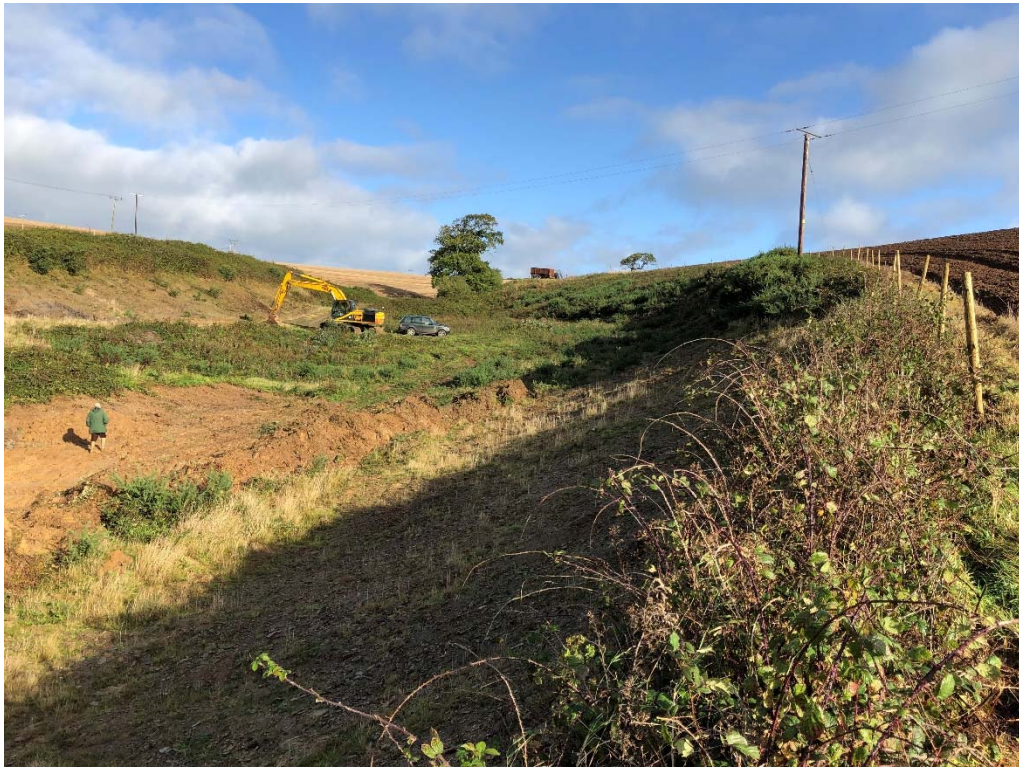
Photograph 11: View of deposition area, looking in a northerly direction. [01 October 2019].
