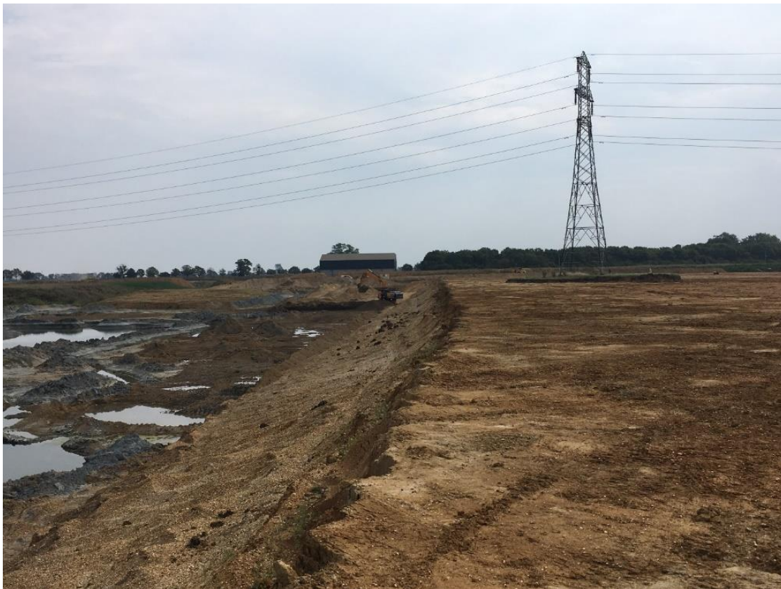
Figure ESID1: Working face with Active Extraction Area (left) and Soil Stripping Area (right)
