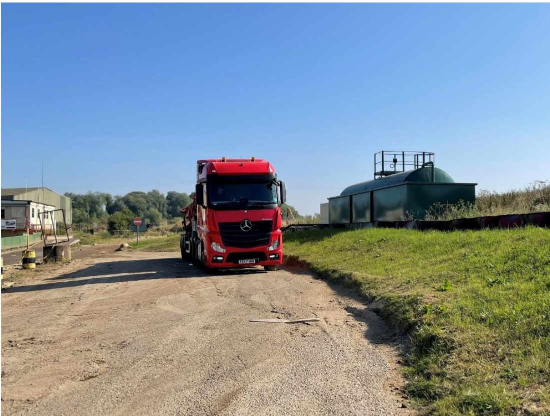
Figure ESID3: Road Tanker in Loading Bay and Leachate Storage Tank (to be retained)
