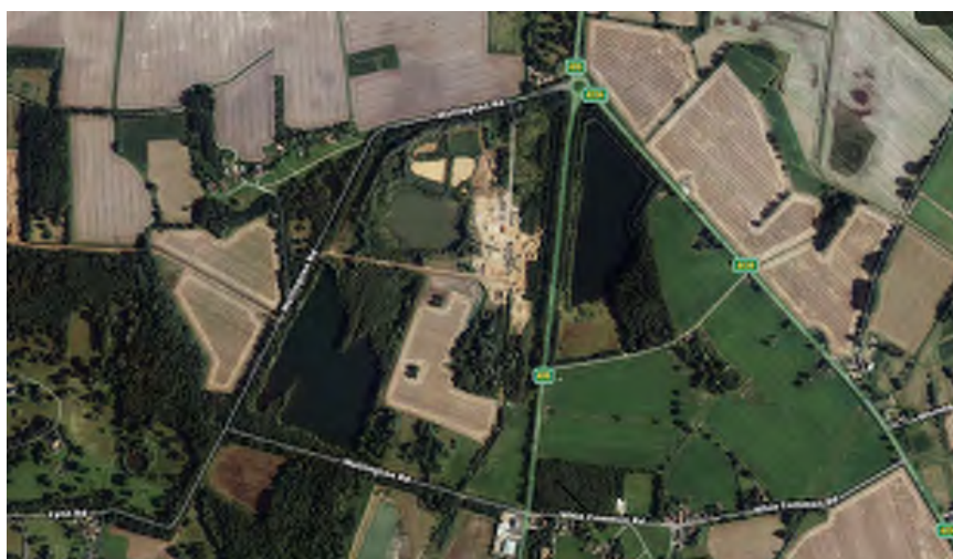
Figure 002: Existing Site Layout – Aerial Photograph
