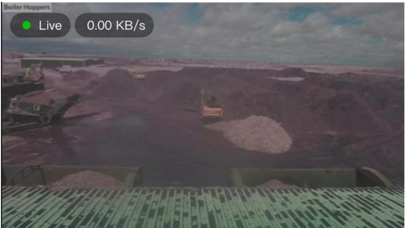
Figure 6-1: Biomass feed hoppers
