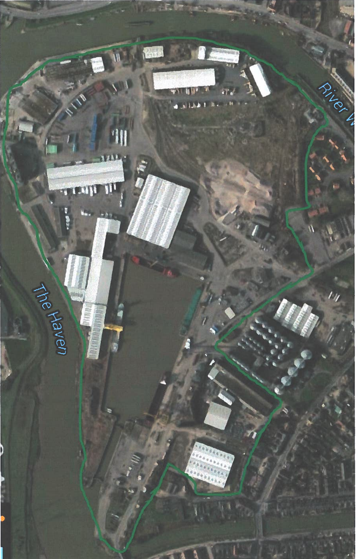
Appendix 2a - Aerial photo of Port of Boston, showing boundary in green PE21 6BN
