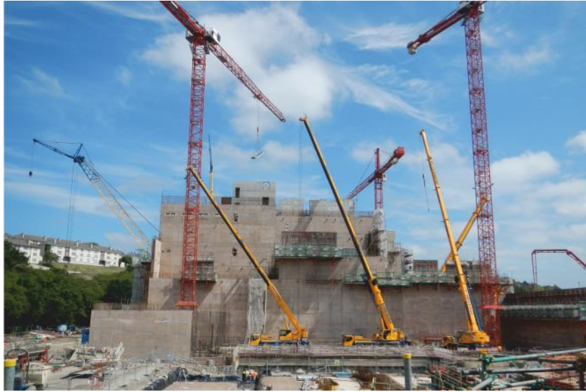
Graphic 3.26: Typical cranes used to construct a EfW CHP Facility
