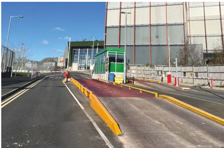
Graphic 3.10: A typical gatehouse/weighbridge
