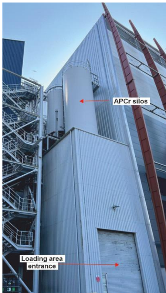
Graphic 3.7: A typical air pollution control storage silos and loading entrance
