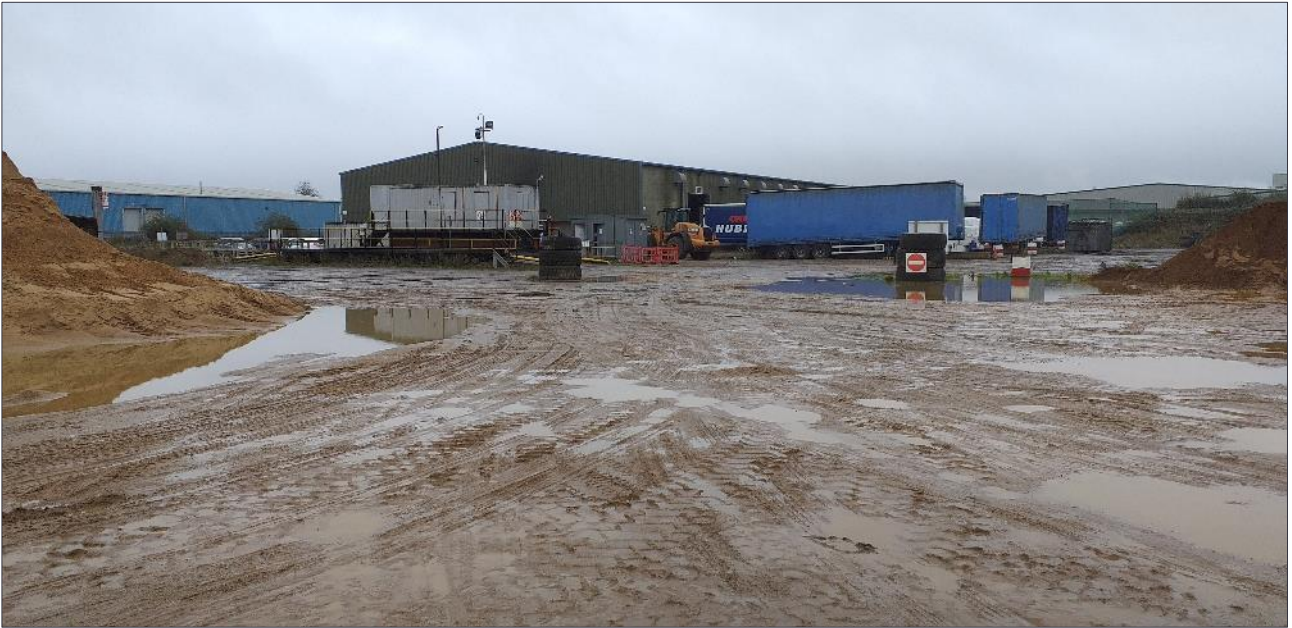
Looking north-east from the north-west quadrant towards the weighbridge, site cabins and Waste Reception Warehouse (WRW).
