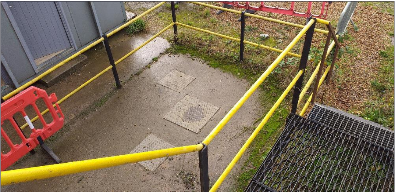
Location of septic tank adjacent to the south-west side of the weighbridge.
