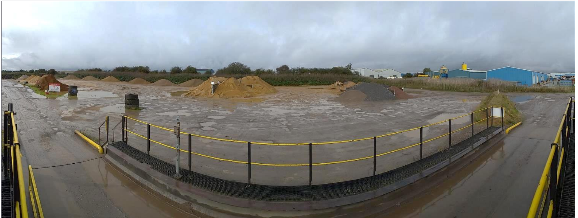
Panorama looking north-west from the site Weighbridge. Overlooking the aggregate storage area and the adjacent concrete products manufacturing site (blue) to the left.
