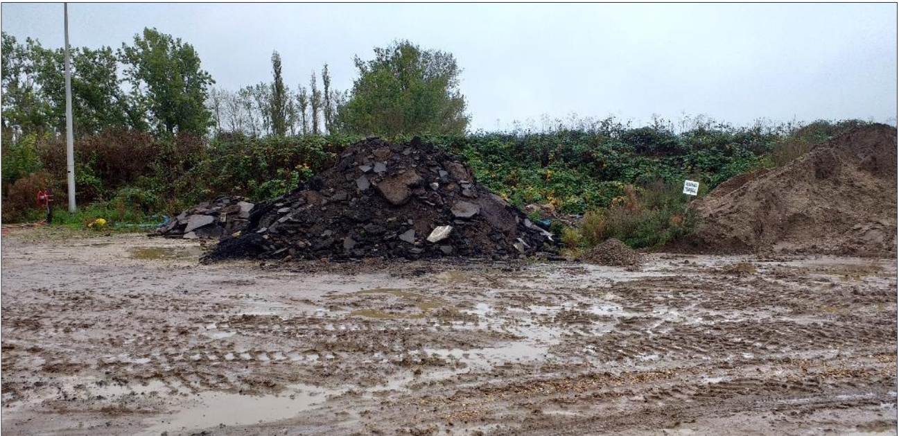
Looking south from the south-east quadrant of Area A. Stockpiles of road scalplings (left) and screened topsoil (right).
