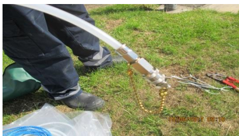
Air release valve connected
