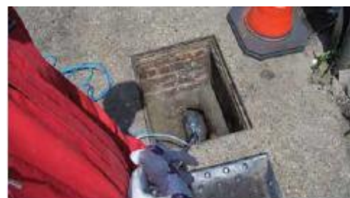
Connect white hose to pump insert bladder in drain and pump up Pump and hose connection
