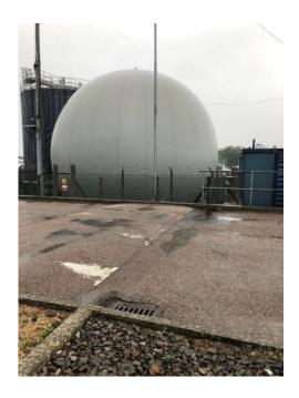
Photo of one of the three Secondary Digesters on site. Digested sludge is transferred to the digested sludge dewatering belts.
