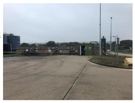
Photo of the Sludge Buffer Tank. This receives blended indigenous and imported sludges, which are pumped to one of the four Primary Digesters on site.
