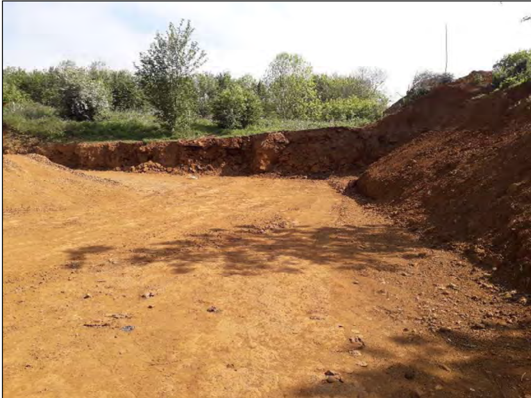
Typical condition of excavation boundary (view of northeastern corner and
