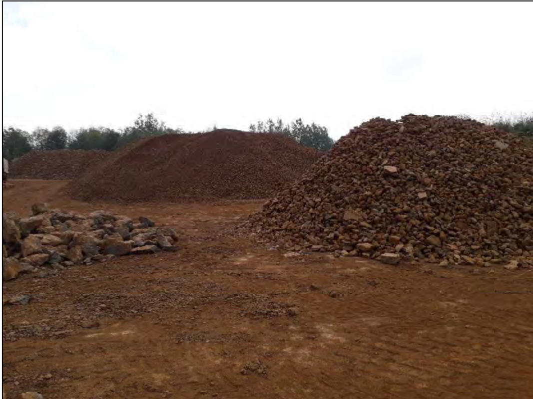
Stockpiles of screened materials in centre of site
