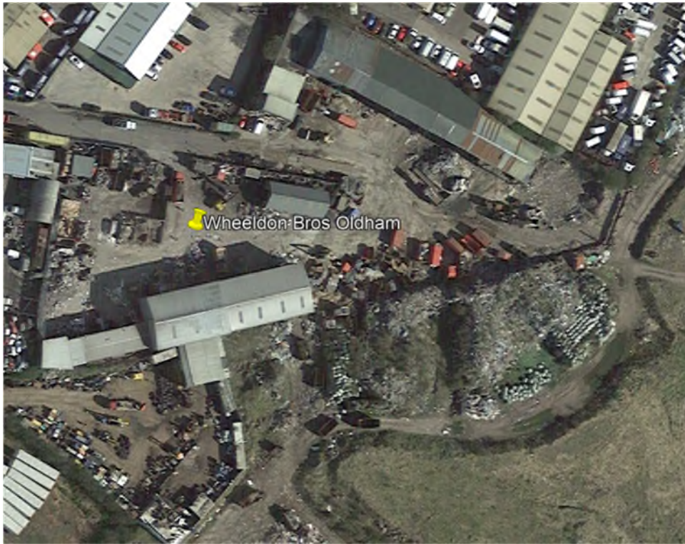
2021 - site taken over by WB and cleared of waste, perimeter fence erected. Similar to present day. Off-site waste deposits to the south still in situ and are still in place in 2023 at the time of writing.
