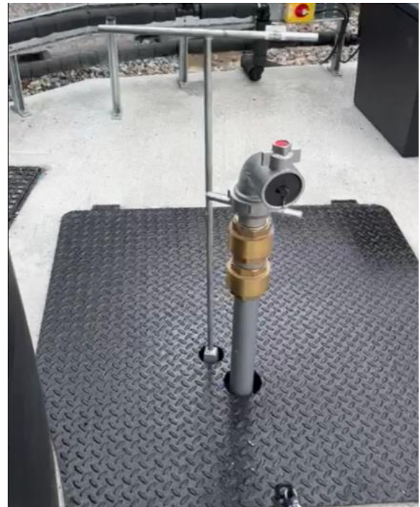
Purpose built discharge point
