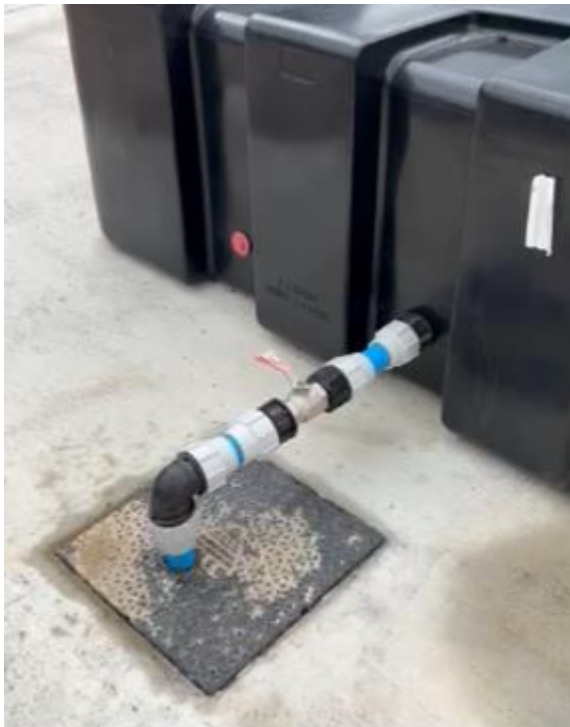
Discharge point to foul sewer
