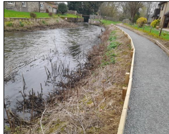
Photograph six: View looking towards the Turf Lock (along the right bank)
