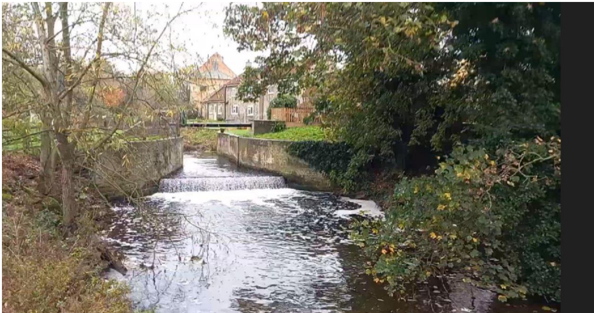
Figure 2-1 Photograph of upstream end of Turf Lock captured from the downstream true right bank on 15/11/2022.
