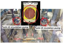
First find out which tank (12/13) is leaking, after that switch "off" the circulation pump of the anodising tank. PPE must be worn while doing this work
