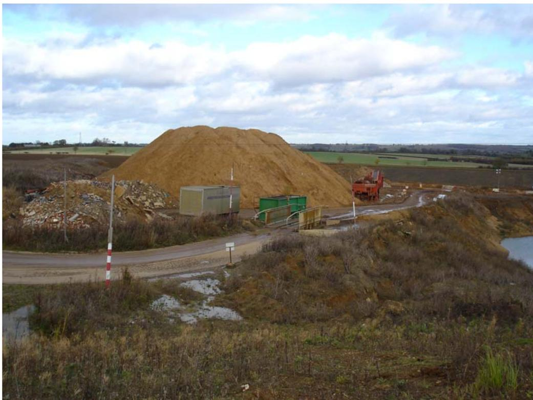
**Photo 2** – View to NNE from SW corner of site. The internal haul road and wheelwash facility are evident in the middle of the photograph; the engineered side wall of Cell 5 is evident in the right back ground.
