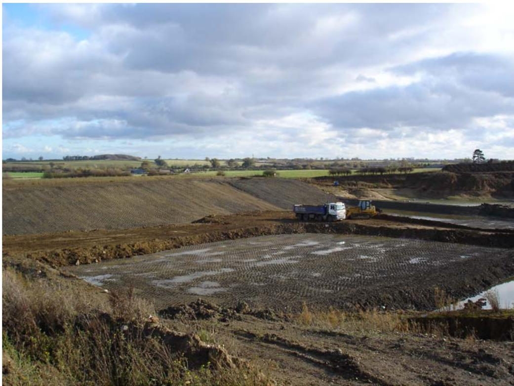
**Photo 4** – View to SE from NW corner of the current active cell (Cell 5) showing landfilling with soils and stones. The engineered basal liner and side wall construction of the Cell are evident, with the intracell bund in the background.
