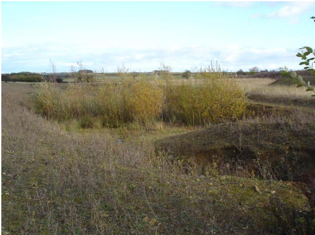
**Photo 10** – Western boundary of the lagoons of the surface water management system. The input of the drainage channel is evident in the foreground; the first lagoon is evident, which is heavily vegetated with willow trees and rushes.
