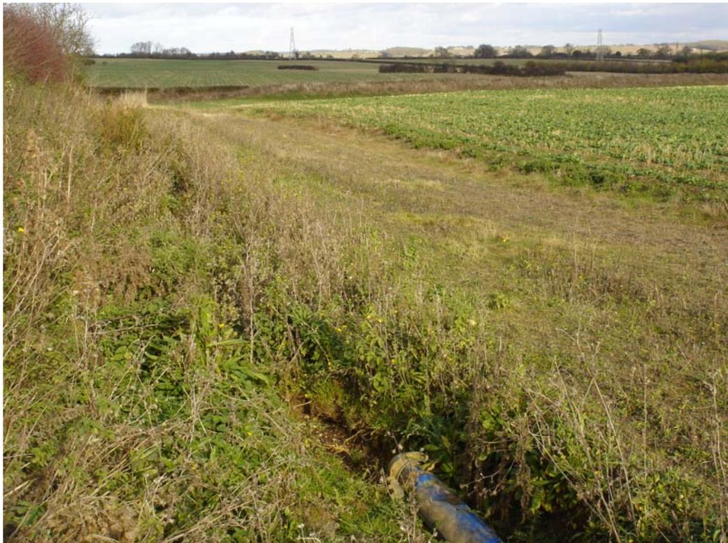
**Photo 8** – Drainage channel to the east of the landfill area, which channels drainage from the site towards the lagoons of the surface water management system.
