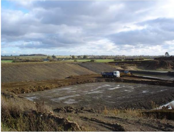
Figure 2.17: Cell 5 engineered basal liner and side wall. Intracell bund in background.
