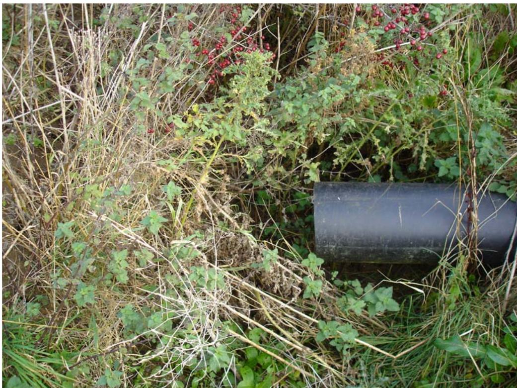
**Photo 14** – Consented discharge point for surface water drainage from the site.
