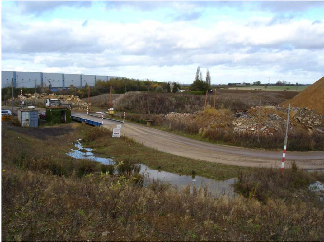
**Photo 1** – View to NNW from SW corner of site, showing site entrance, amenity area and weighbridge (left, middle ground) and internal haul road (middle ground). The restored areas of the Site are evident in the right back ground.
