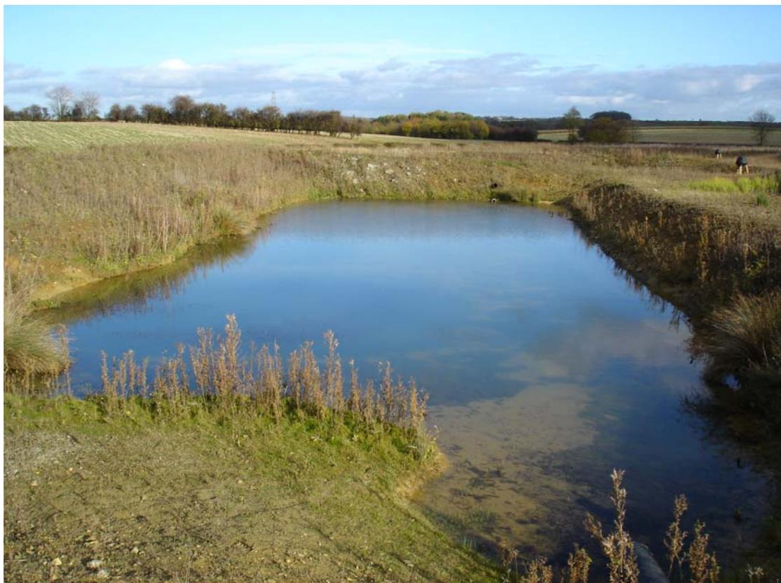
**Photo 12** – View to ENE across the second drainage lagoon. The discharge into from the western lagoon was visually estimated to be about 1 litre/min.
