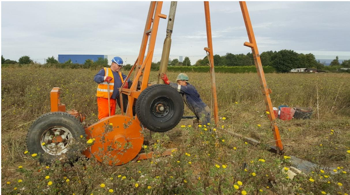
**Plate 2 – Installation of gravel down borehole**
