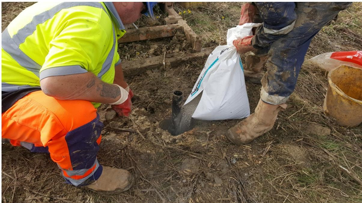
**Plate 4 – Metal protective casing secured in place by concrete around top of standpipe**
