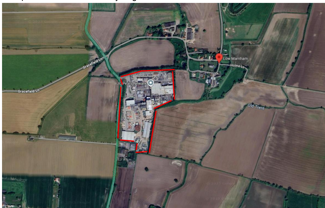
Satellite view of the JG Pears facility, Low Marnham, Newark
