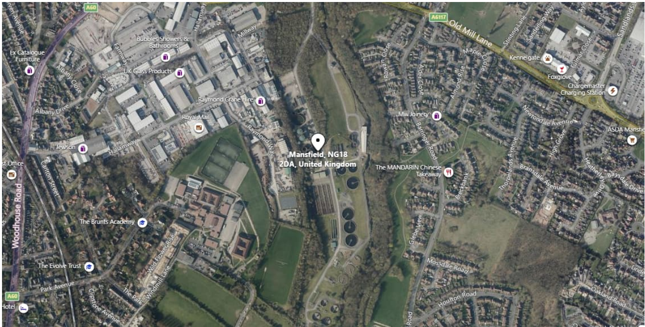
Figure i Aerial view of Mansfield Sewage Treatment Works
