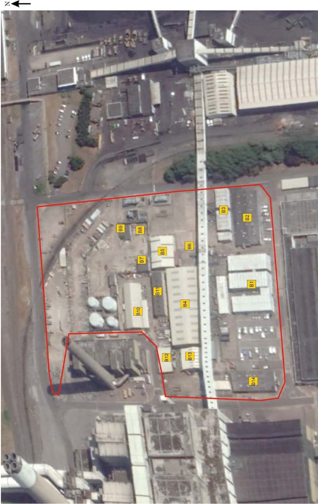
Figure 2a: Survey Area 1
