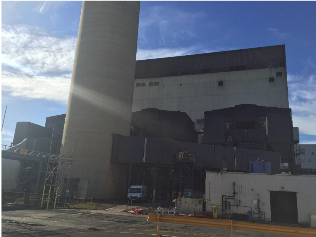
Figure 4: Electrostatic Precipitators (Boiler House Rear, ESPs and Stack Ductwork)
