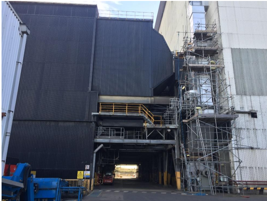
Figure 1: Electrostatic Precipitators (Unit 1 A0 & B0 Fields – Boiler House Visible to Right)
