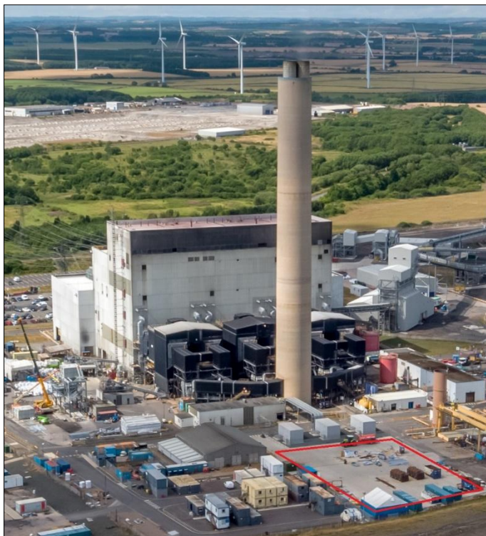
Figure 11: Potential location for Low-Dust SCR (Red Boundary)
