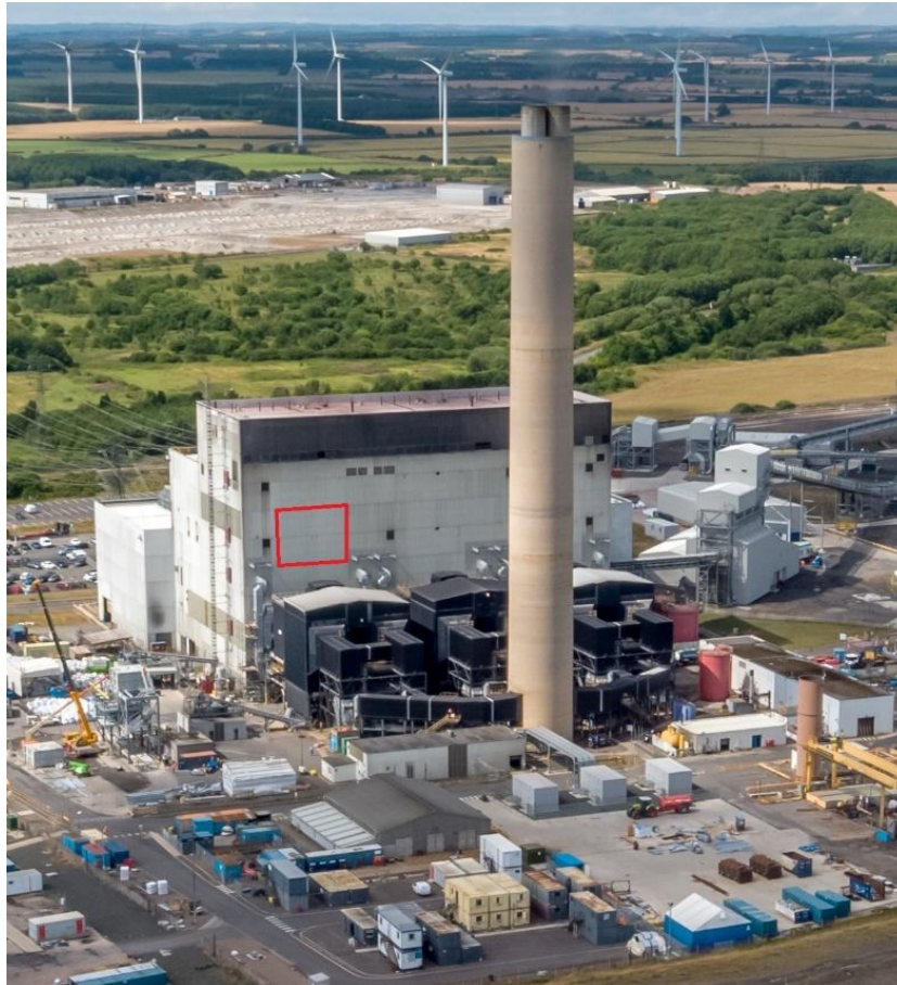
Figure 10: Indicative location of new ductwork/SCR for high dust option [Unit 3 shown, other units identical]
