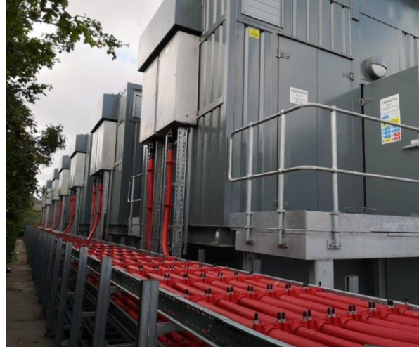
Photograph 3 – Ground Floor Excool Units
