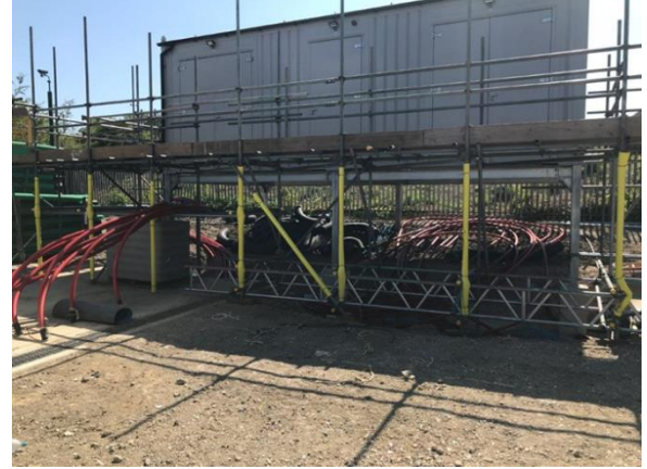
Photograph 8 – London Energy Substation
