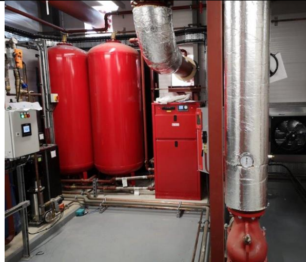
Photograph 5 – Chiller Pumps and Vessels
