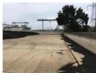
Photo showing Post Digestion Dewatering plant (left photo) and general size of the Cake Pad (bottom photos). Dewatered digested sludge cake is transferred to the Cake Pad area via conveyors and stored prior to removal from site.
