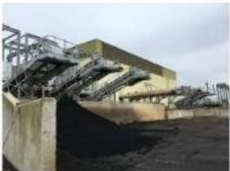
Photo showing Post Digestion Dewatering plant (left photo) and general size of the Cake Pad (bottom photos). Dewatered digested sludge cake is transferred to the Cake Pad area via conveyors and stored prior to removal from site.
