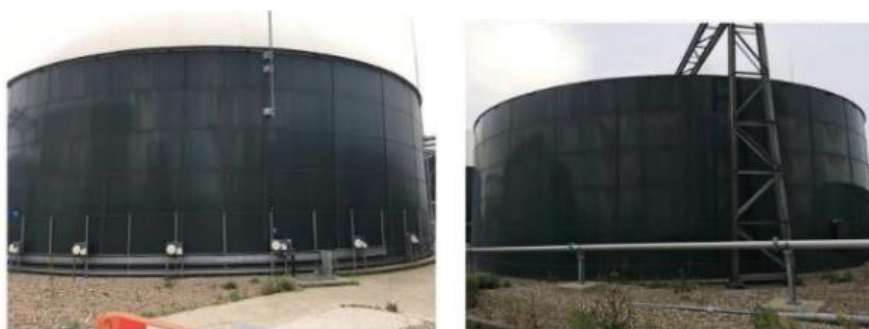
Photo showing one of the four Secondary Digester Tanks (SDTs) and the Post Digestion Dewatering Feed Tank. Digested sludge is received from the SDTs and pumped to the Post Digestion Dewatering Feed Tank and the Post Digestion Dewatering plant.
