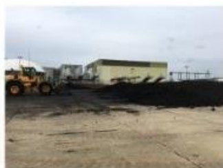
Photo showing Post Digestion Dewatering plant (left photo) and general size of the Cake Pad (bottom photos). Dewatered digested sludge cake is transferred to the Cake Pad area via conveyors and stored prior to removal from site.
