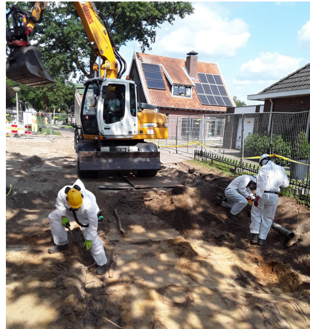
Removing asbestos contaminated soil | NTP
