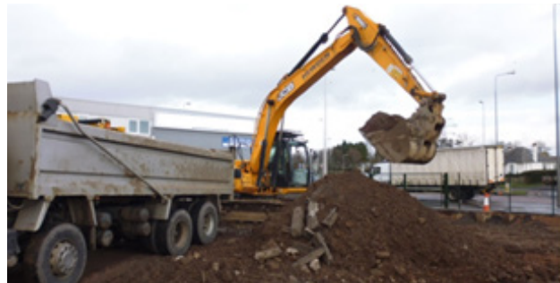
Typical remediation earthworks activities in UK | AECOM
