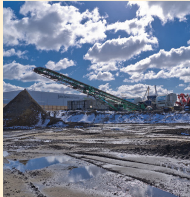
Processing plant | John F Hunt
