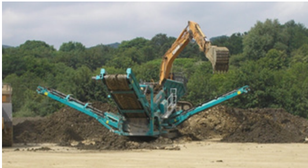
Mechanical screening of excavated soil | AECOM
