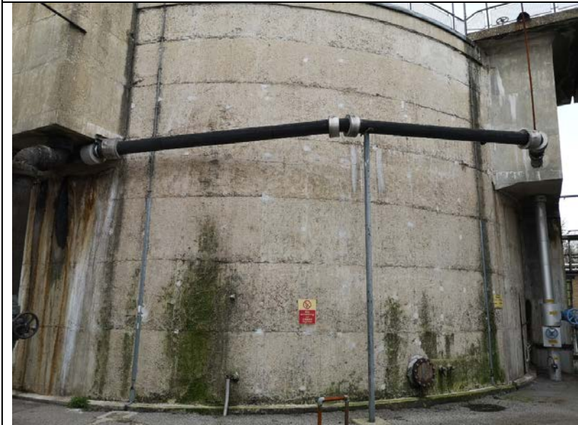
Condition of digester
