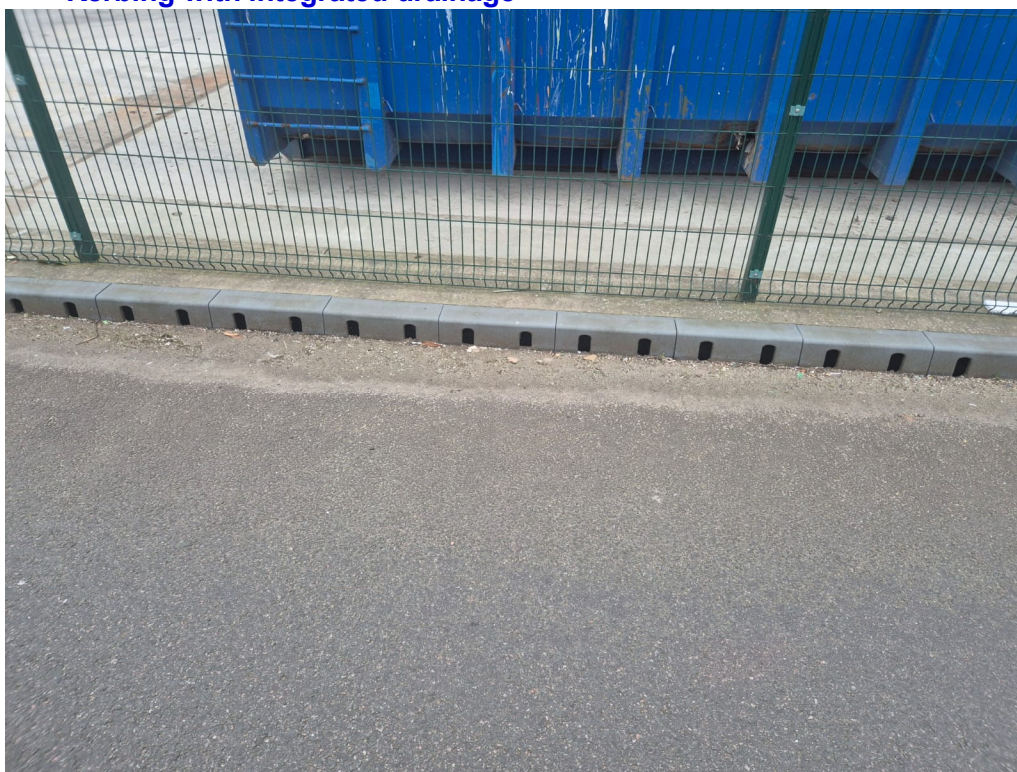
Figure 8 Kerbing with integrated drainage
