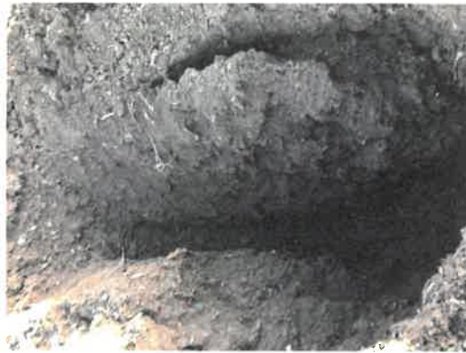
Pile 5 S2 Collapse.
