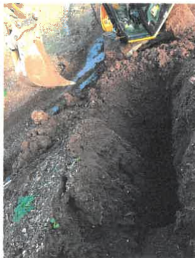
Pile 5 S1 Collapsed side after excavation.
