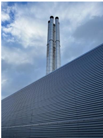
Figure 13: Boiler exhaust stacks exiting the building
