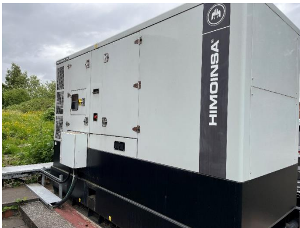
Figure 37: 1 x .0.367 MWth standby generator (Ref GEN16)
