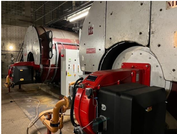
Figure 11: 2 x 7.143 MWth boilers (Ref A07-1 & A07-2)
