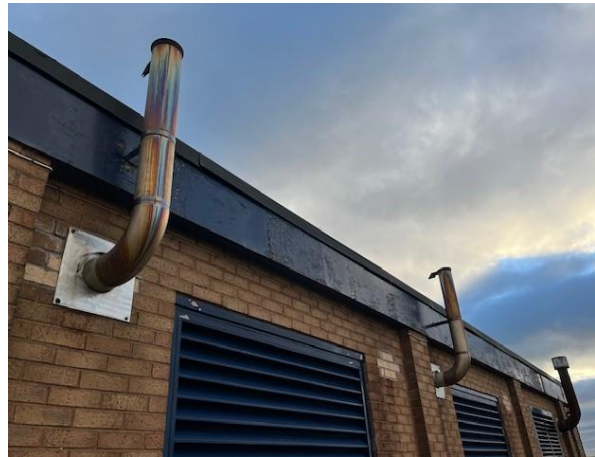
Figure 31: GEN06 & GEN07 vertical capped exhaust stacks exiting the building
