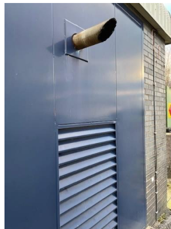
Figure 44: GEN23 horizontal exhaust stack exiting the building
