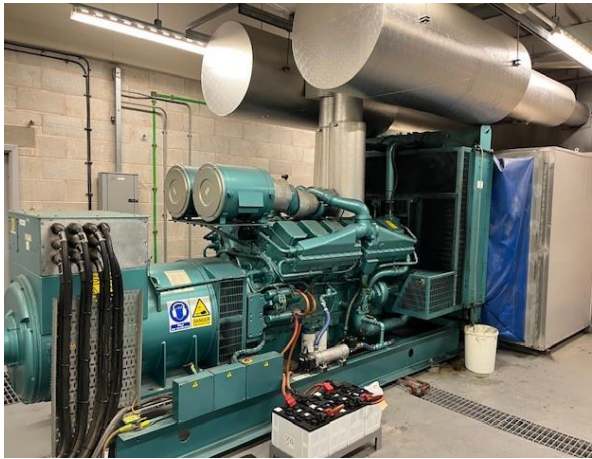
Figure 40: 1 x .2.424 MWth standby generator (Ref GEN21)
