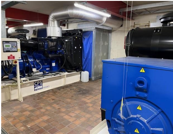
Figure 30: 2 x 1.333 MWth standby generator (Ref GEN06 & GEN07)
