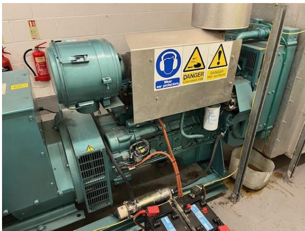
Figure 43: 1 x .0.285 MWth standby generator (Ref GEN23)
