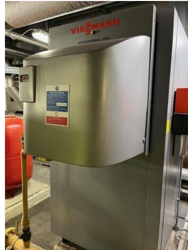
Figure 9: 1 x 0.577 MWth boilers (Ref A05-2)
