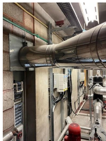
Figure 15: Shared exhaust exiting the boiler room
