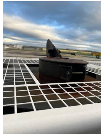
Figure 33: GEN09 vertical capped exhaust stack
