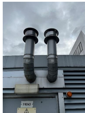
Figure 20: Vertical capped stacks exiting the building
