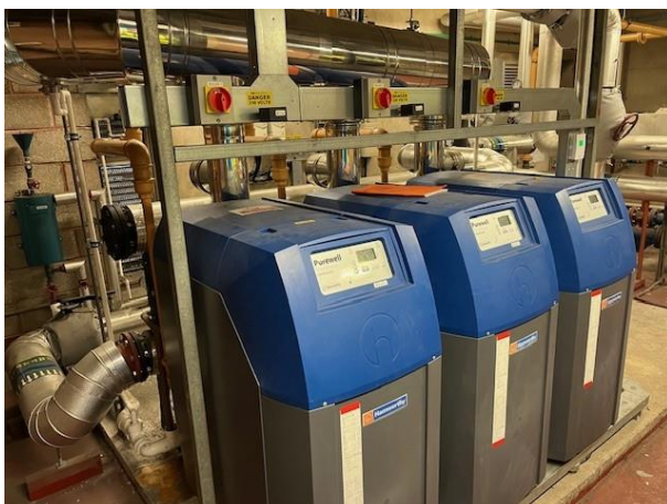
Figure 14: 3 x 0.1752 MWth boilers (Ref A11-A, A11-B & A11-C)
