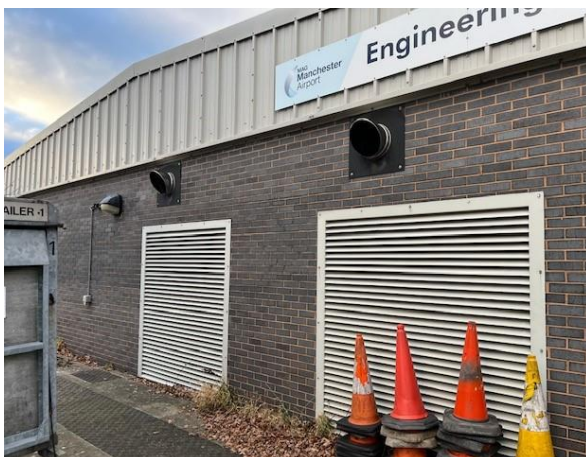
Figure 29: GEN04 & GEN05 horizontal exhaust stacks exiting the building
