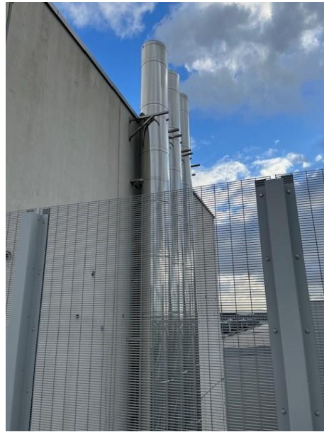
Figure 22: Vertical exhaust stacks exiting the MAN - TP Energy Centre
