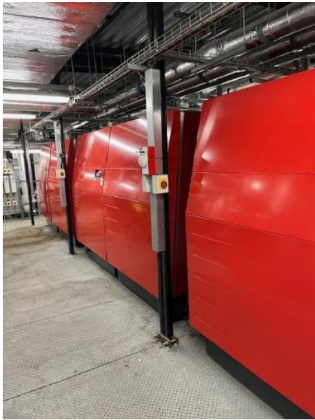
Figure 21: 3 x 2.144 MWth boilers (Ref A24-1, A24-2 & A24-3) and 1 x 0.558 MWth boiler (Ref A24-4)
