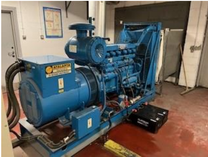
Figure 48: 1 x .0.800 MWth standby generator (Ref GEN27)
