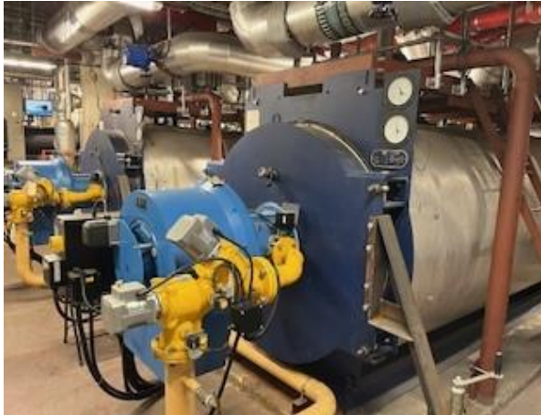
Figure 1: 2 x 4.643 MWth boilers (Ref A01-A & A01-B)
