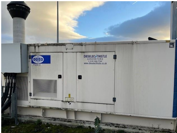
Figure 32: 1 x 1.333 MWth standby generator (Ref GEN09)
