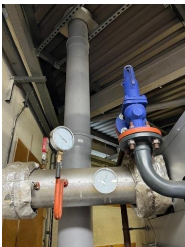
Figure 10: Boiler exhaust exiting the boiler room
