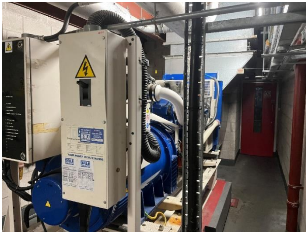
Figure 54: 1 x .1.828 MWth standby generator (Ref GEN31)
