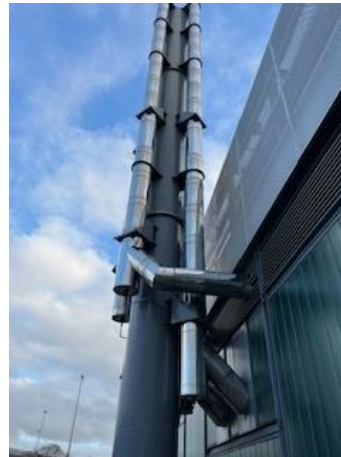
Figure 7: Boiler exhaust stacks exiting the boiler room
