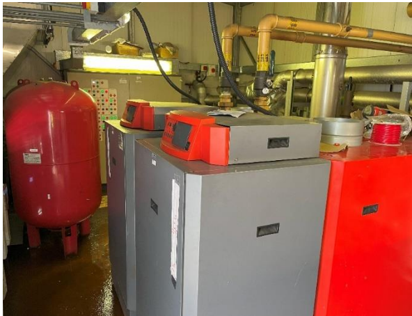
Figure 3: 3 x 0.673 MWth boilers (Ref A02-1, A02-2 & A02-3)
