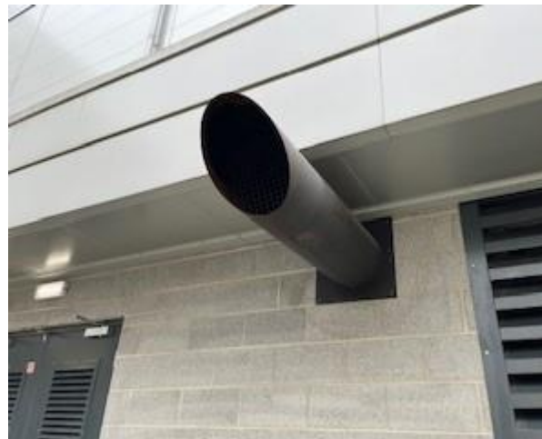
Figure 51: Horizontal exhaust stack for GEN29 exiting the building
