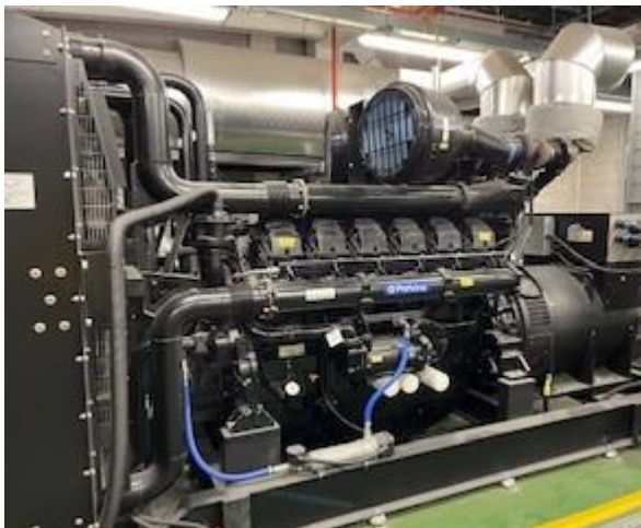
Figure 50: 1 x .4.000 MWth standby generator (Ref GEN29)
