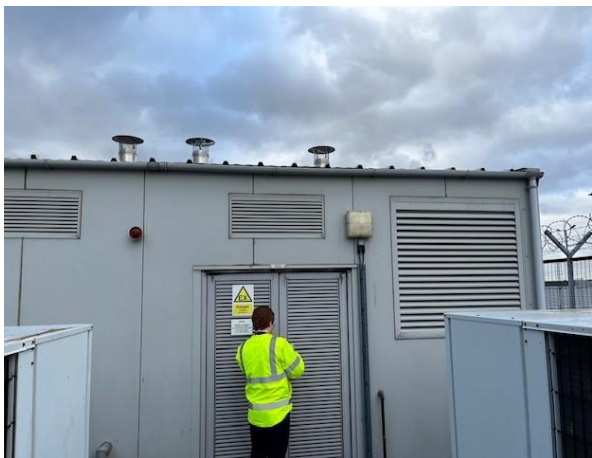
Figure 5: Vertical capped stacks
