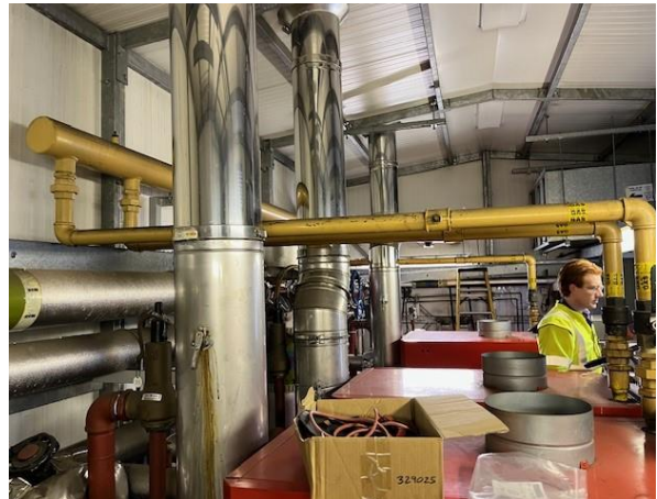
Figure 4: Boiler exhausts exiting the boiler room
