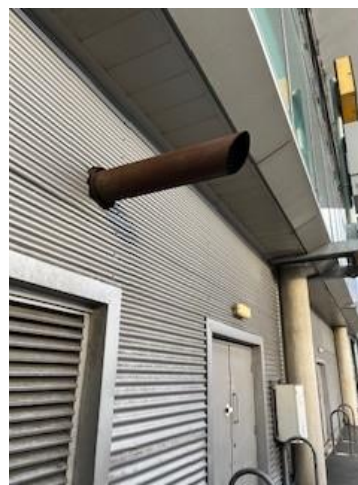
Figure 35: GEN11 horizontal exhaust stack exiting the building
