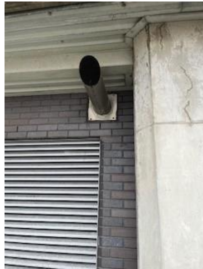
Figure 49: Horizontal exhaust stack for GEN27 exiting the building
