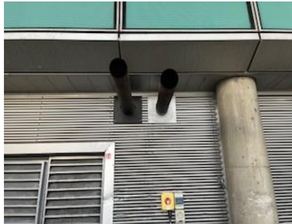
Figure 53: Twin horizontal exhaust stacks for GEN30 exiting the building
