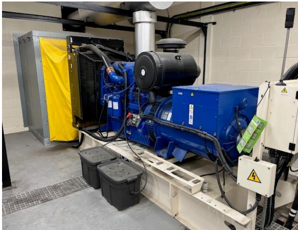
Figure 27: 1 x 1.333 MWth standby generator (Ref GEN04)
