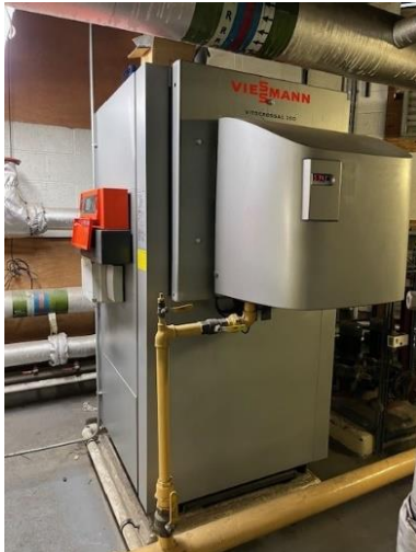
Figure 8: 1 x 0.577 MWth boiler (Ref A05-1)
