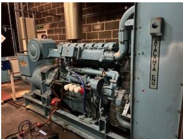
Figure 34: 1 x 1.212 MWth standby generator (Ref GEN11)
