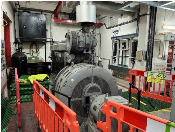
Figure 36: 1 x .0.830 MWth standby generator (Ref GEN12)
