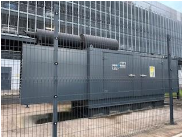
Figure 25: 1 x 0.848 MWth standby generator (Ref GEN01)
