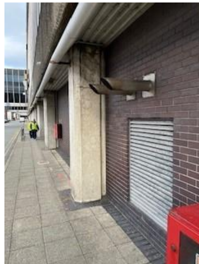
Figure 47: Twin horizontal exhaust stacks for GEN26 exiting the building
