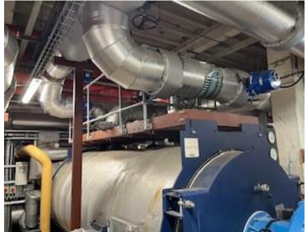
Figure 2: Boiler exhausts exiting the boiler room
