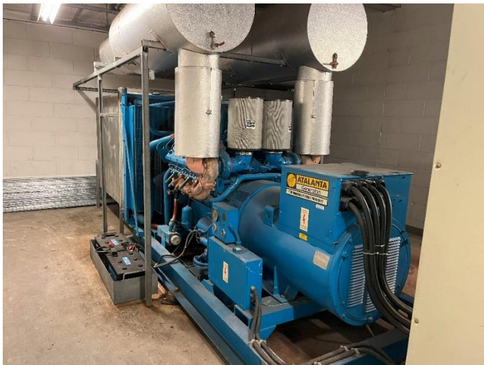
Figure 46: 1 x .0.985 MWth standby generator (Ref GEN26)
