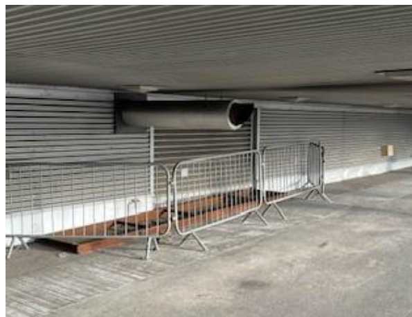
Figure 39: GEN19 horizontal exhaust stack exiting the building
