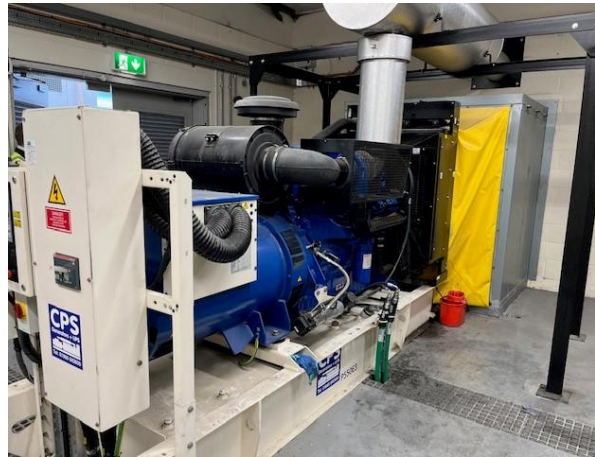
Figure 28: 1 x 1.333 MWth standby generator (Ref GEN05)
