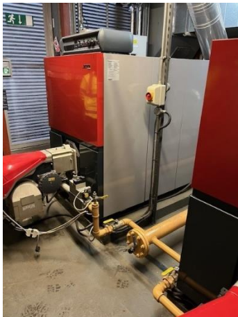
Figure 17: 2 x 0.714 MWth boilers (Ref A13-1 & A13-2)
