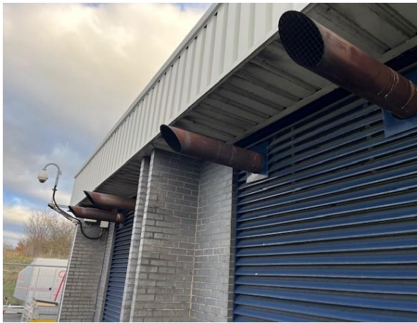
Figure 42: GEN21 & GEN22 horizontal twin exhaust stacks exiting the building
