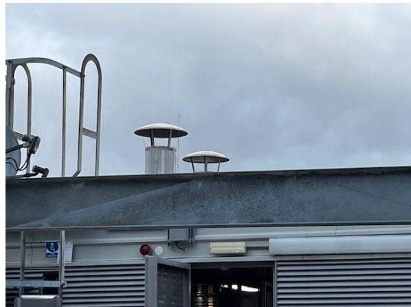
Figure 18: Vertical capped stacks exiting the building
