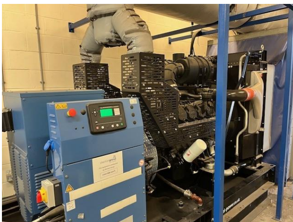
Figure 55: 1 x .1.333 MWth standby generator (Ref GEN32)
