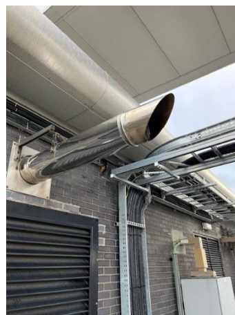
Figure 56: Horizontal exhaust stack for GEN32
