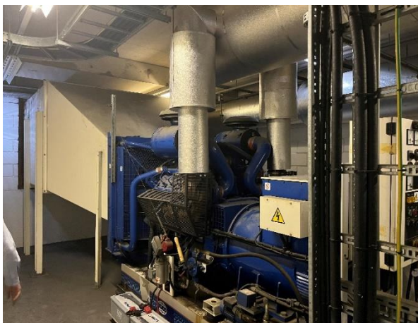
Figure 38: 1 x .1.212 MWth standby generator (Ref GEN19)
