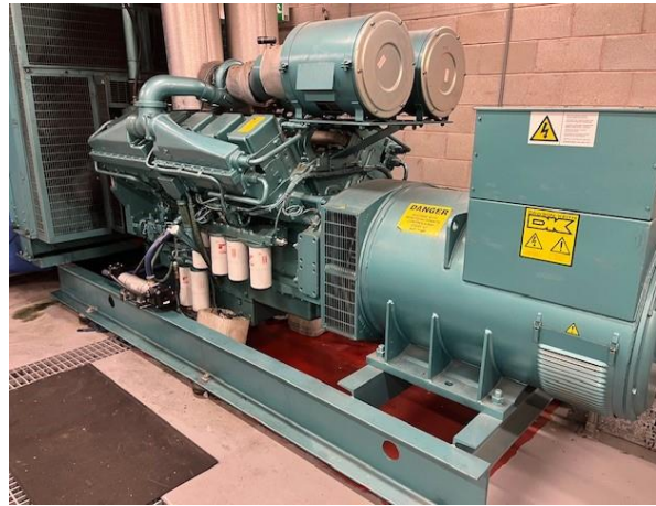
Figure 41: 1 x .2.424 MWth standby generator (Ref GEN22)
