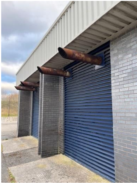
Figure 45: Twin horizontal exhaust stacks for GEN24 & GEN25 (although not pictured, generator type are identical to GEN21 & GEN22)
