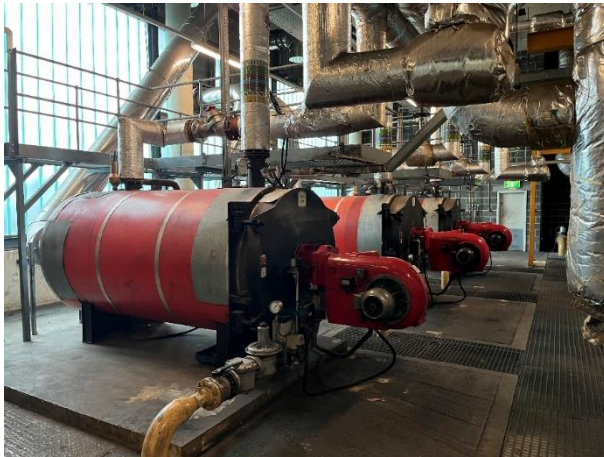
Figure 6: 3 x 2.857 MWth boilers (Ref A03-1, A03-2 & A03-3)
