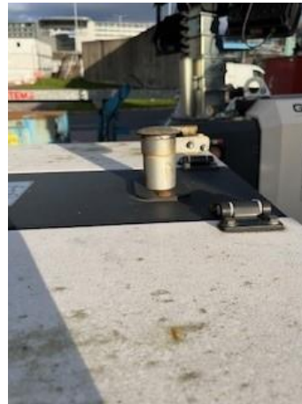
Figure 58: Vertical capped exhaust stack
