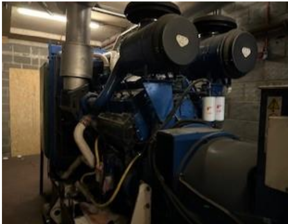
Figure 52: 1 x .1.636 MWth standby generator (Ref GEN30)
