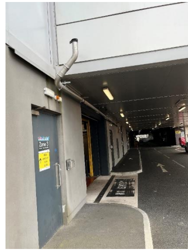
Figure 61: FIR09 vertical stack exiting the building
