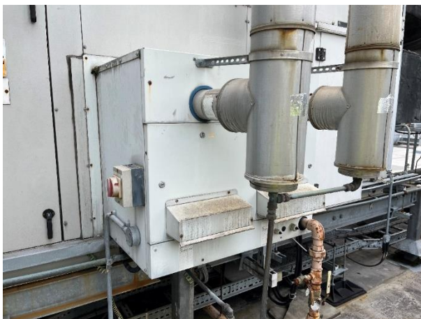
Figure 19: 2 x 0.183 MWth boilers (Ref A17-A & A17-B)
