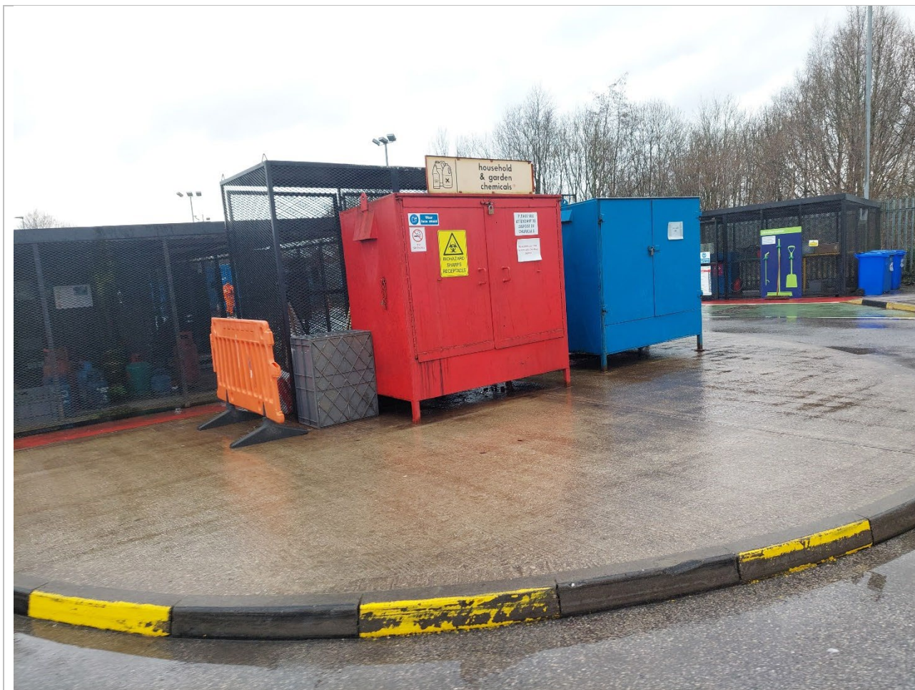
Photograph showing the chemical storage containers looking towards the electricals (WEEE) cage (this section of boundary is unchanged in the proposed permit variation).
