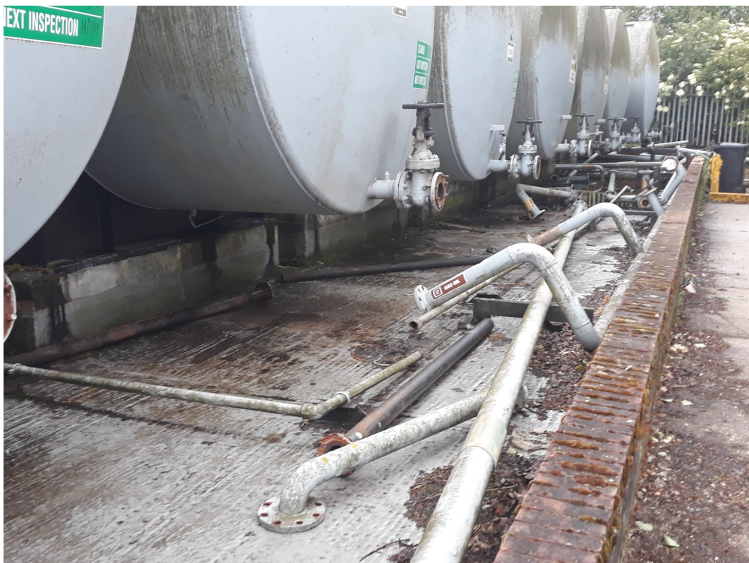
Photo 6— Small brick bund around ASTs.
