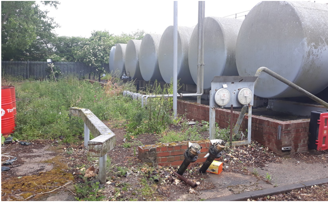
Photo 1—ASTs, with USTs present under soft landscaping.
