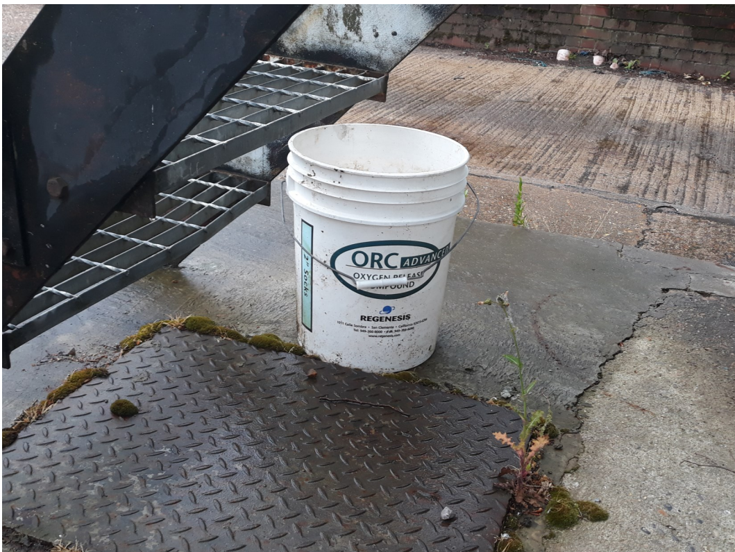
Photo 4— ORC indicating possible former remedial works have taken place.
