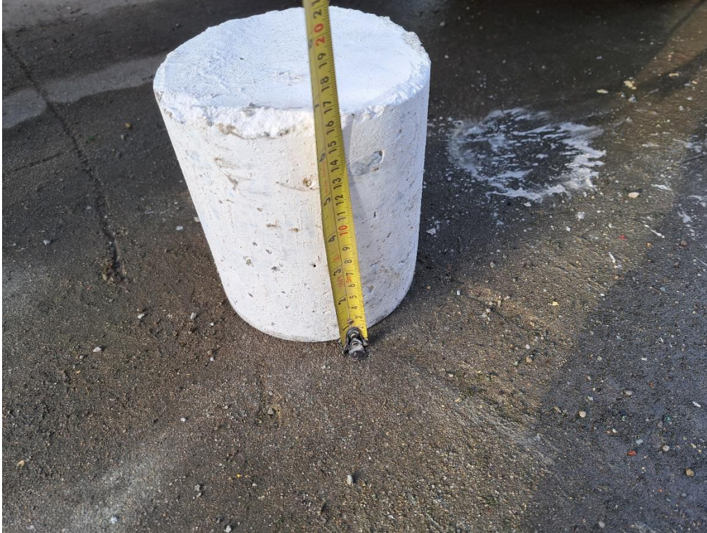
Photograph 3 WS02 detail of concrete core.
