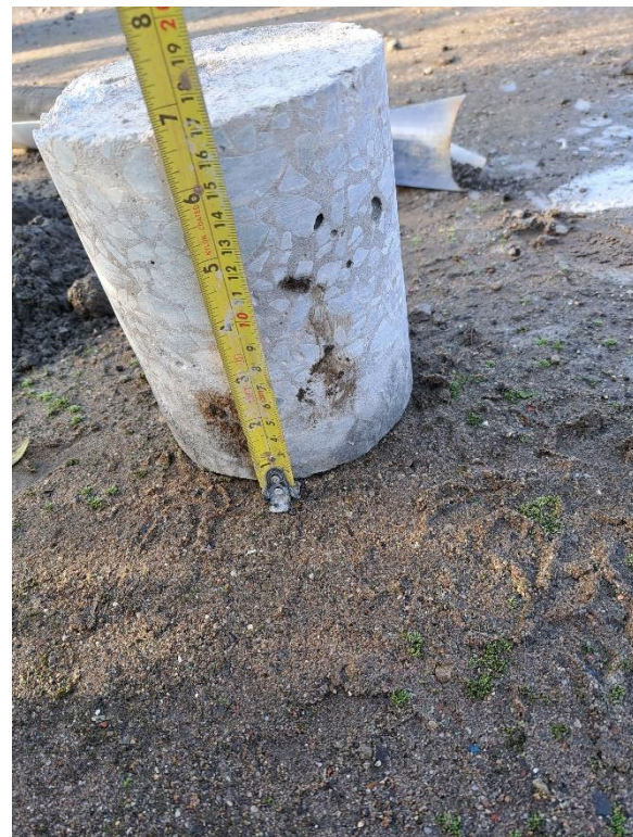
Photograph 2 WS01 detail of concrete core.
