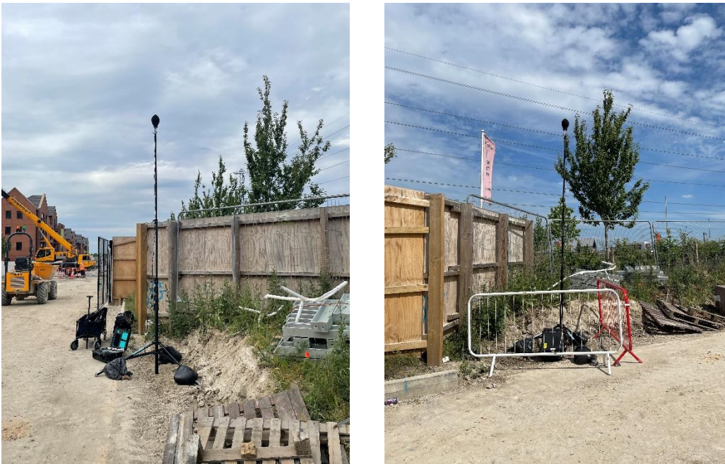
Figure B2: Unattended measurement location L1 (looking north and south respectively)
