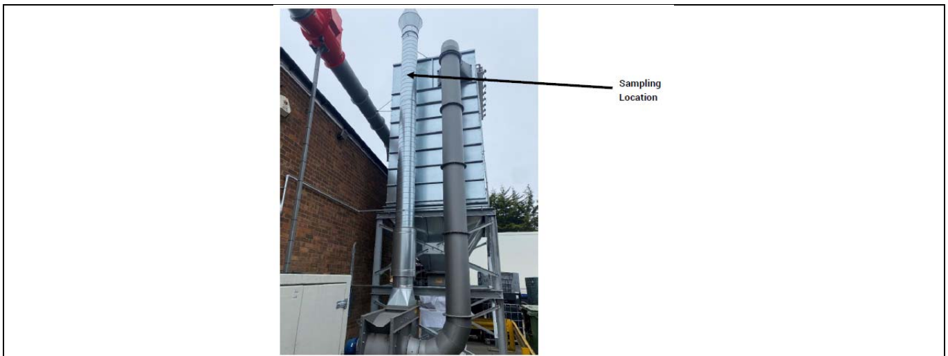
Photo 1: Sampling Location on Stack 1
