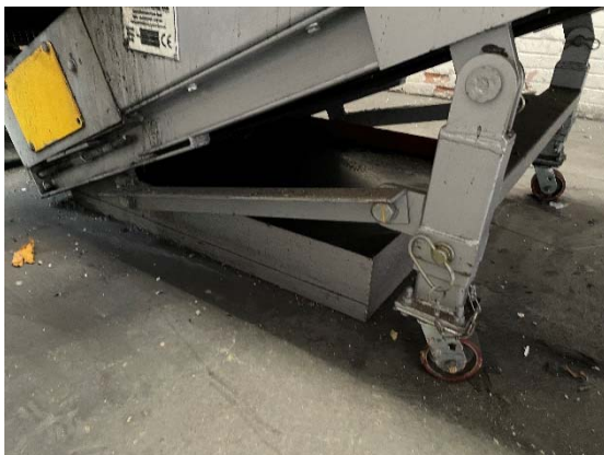
Photo 9: Metal bund to collect any fire water deployed during shredding
