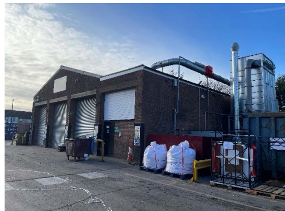
Photo 12: Treatment building, quench tank and emissions stack and abatement
