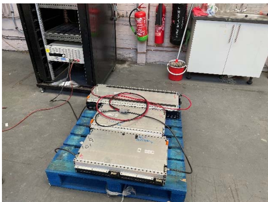
Photo 3: Battery discharge area
