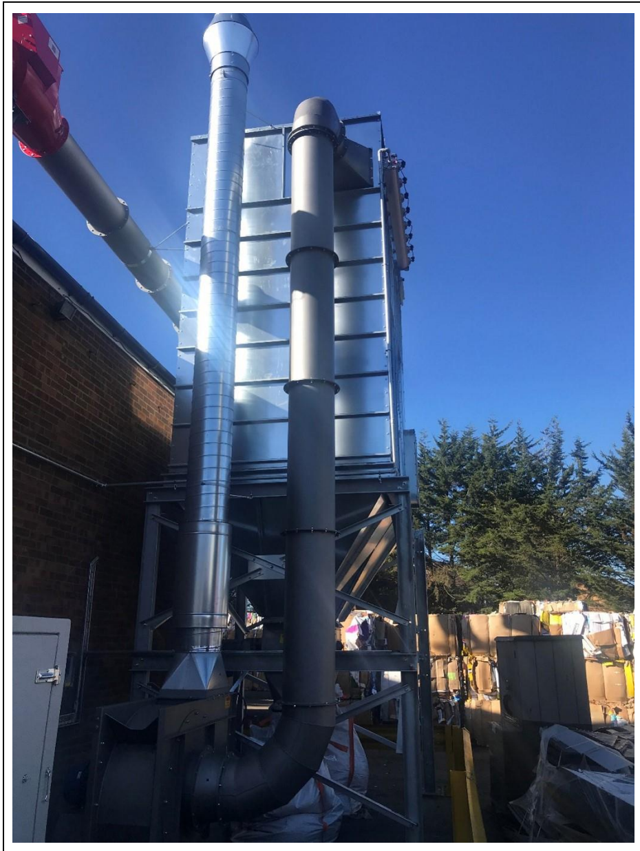
Photograph 3: Dust Extraction Unit including spark detection system (red colour, top left) on inlet piping.
