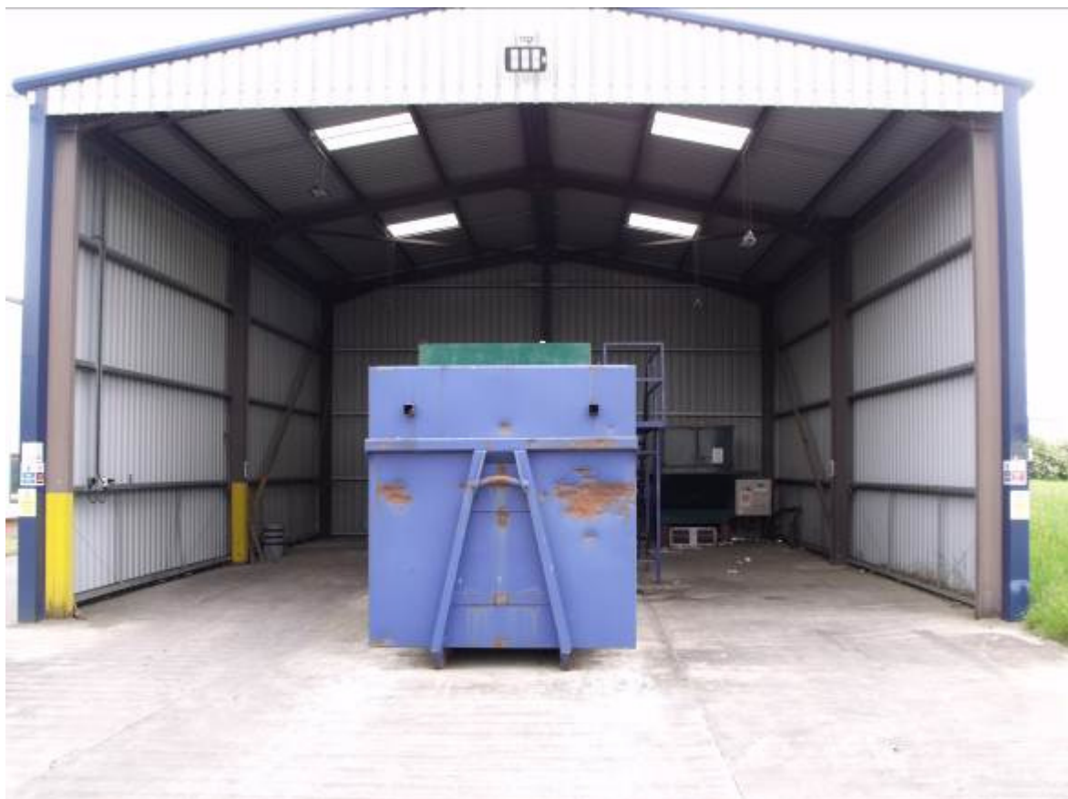
PLATE 6: ALLUMINIUM CLAD PORTAL FRAME SHED HOUSING WASTE SKIP
