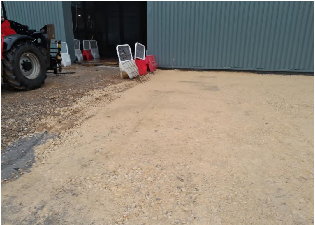
Photo 3 – IBAA removed and replaced with NFS across warehouse vehicle entry
