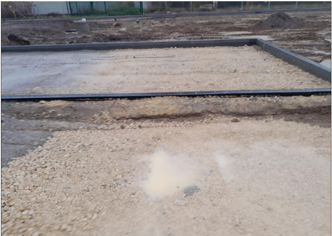
Photo 2 - Eastern zone of removed IBAA, fully replaced with NFS looking to the east.
