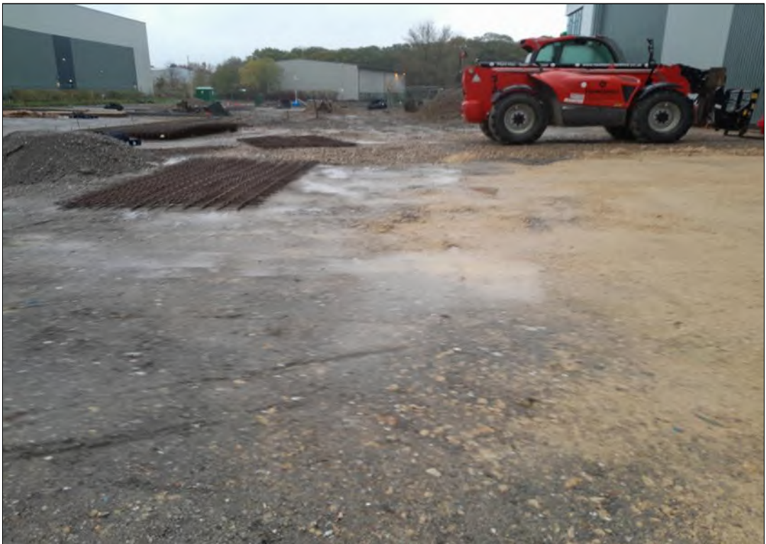
Photo 4 – IBAA and NFS border at this section of the site
